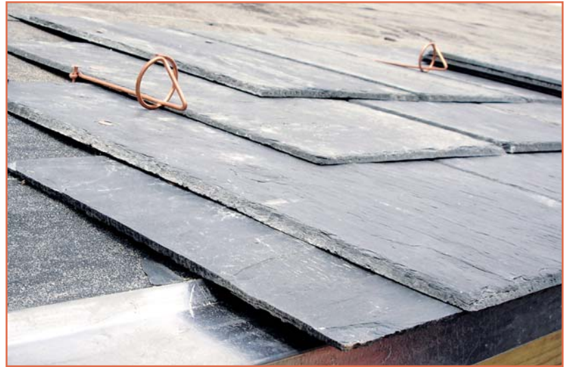
Figure 5 – Copper “loop-the-loop” snow guards are perhaps the least expensive of all snow retention systems. They’re easy to install and effective when used in sufficient quantities.
