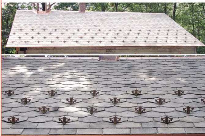
Figure 7 – Polycarbonate snow guards (below) are constructed with durable, UV-resistant plastic and are compatible with all noncopper metal roof systems. They can be attached to a roof with an adhesive or bedded in an adhesive/sealant and mechanically fastened.
