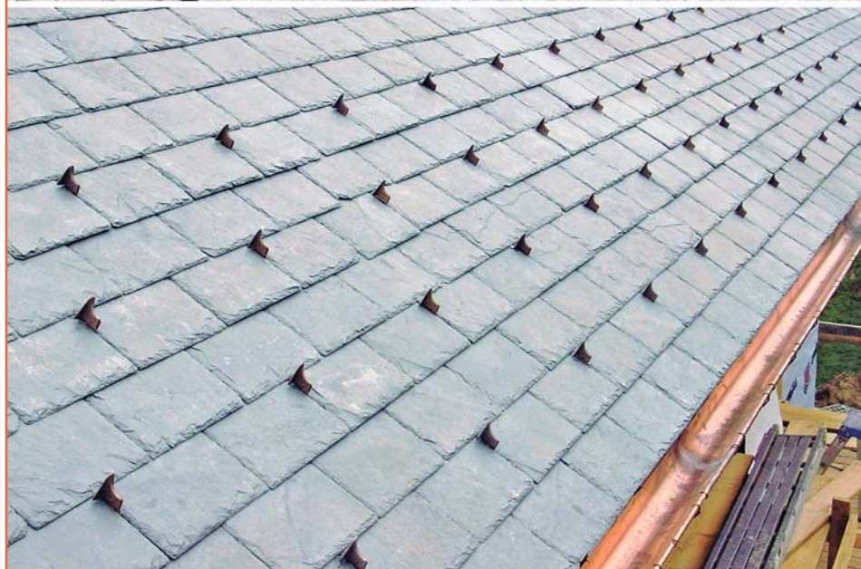
Figure 1 – Mullane's classic 100 and 200 series of snow guards are made from cast bronze and copper. They're available in both standard and retrofit models.
