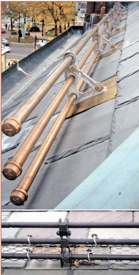
Figure 3 – The Mullane 500 brass and cast-bronze three-pipe snow rail system is one of the strongest snow retention systems available. It can be backed with expanded stainless steel, as shown in the lower portion of this illustration, to catch even small items that may slide off a roof, such as a falling shingle.
