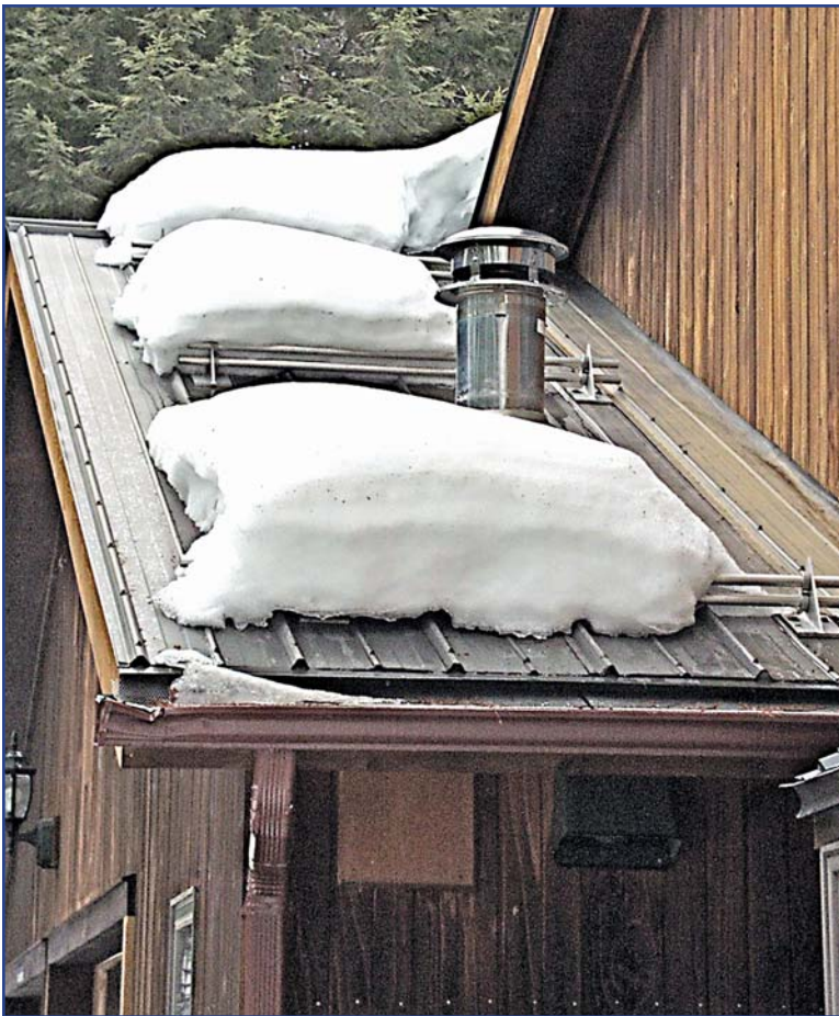
Figure 3 – Pipe-style snow guards create more of a barricade than pad-style snow guards.
