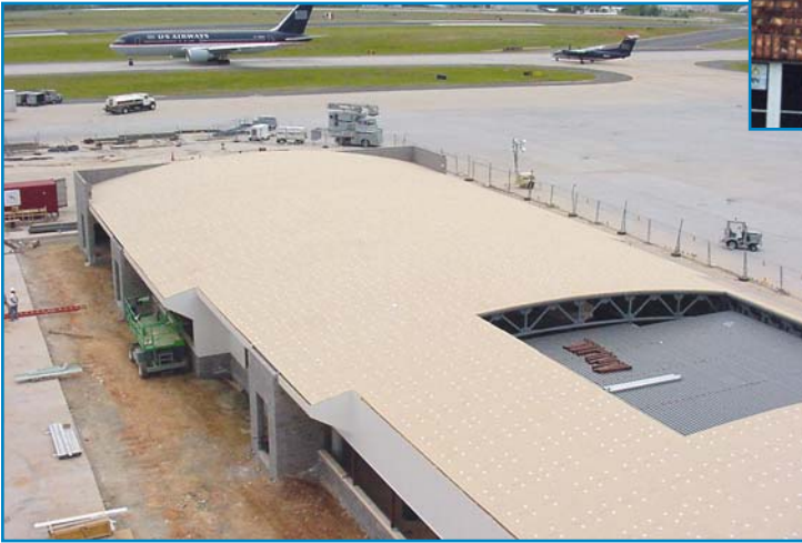
Photo 2 – Loadmaster barrel roof assembly with standing-seam metal on an airport concourse.
