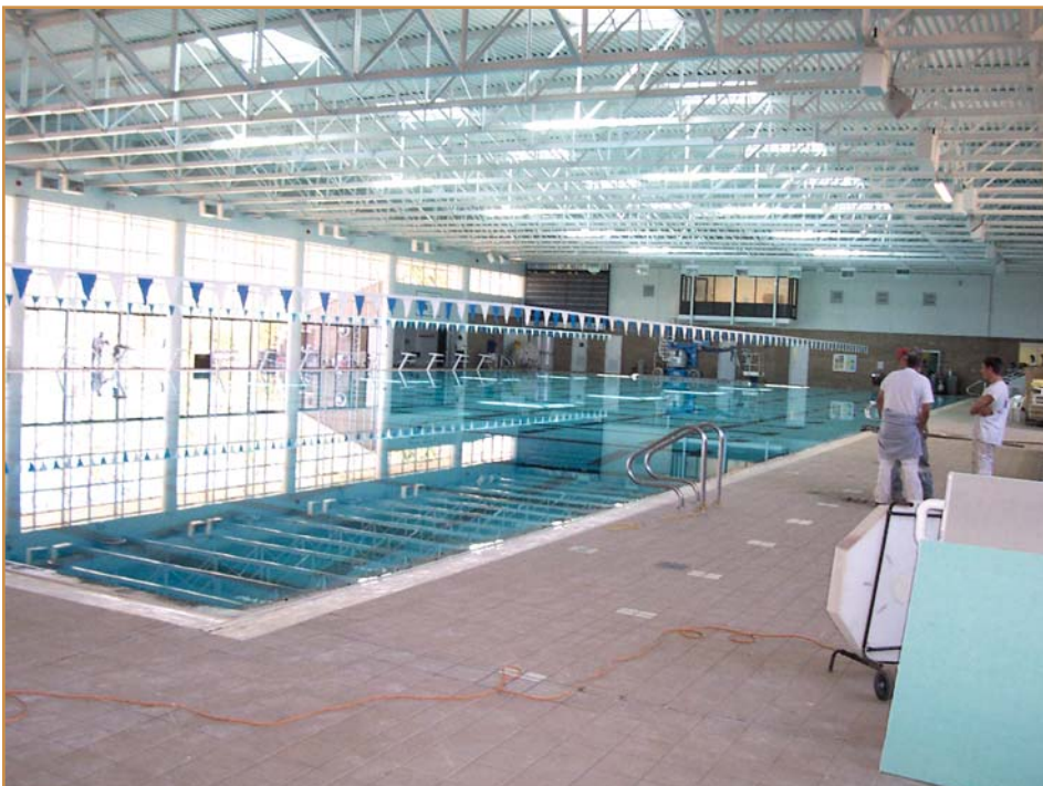
Photo 4 – A corrosion-resistant, FRP roof deck can deliver long, maintenance-free service life in chemical or high-moisture exposures.
