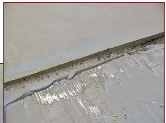
Figure 8 – End-of-the-day cold joint for following day tie-in.
