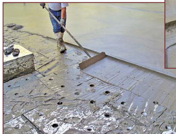
Figure 7 – Cold joint formed using a square aluminum screed.
