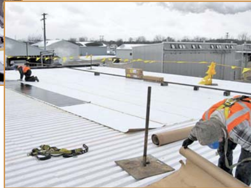
Photo 3 – Mechanical fasteners or cold adhesives are commonly used to attach roofing membrane and insulation to FRP deck.
