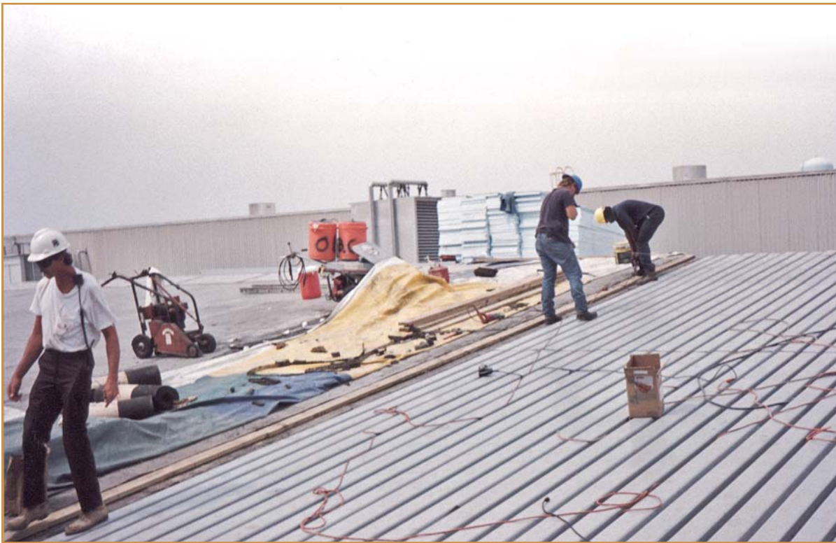
Photo 1 – A corrosion-resistant FRP roof deck can deliver long, maintenance-free service life in chemical or high-moisture exposures.
