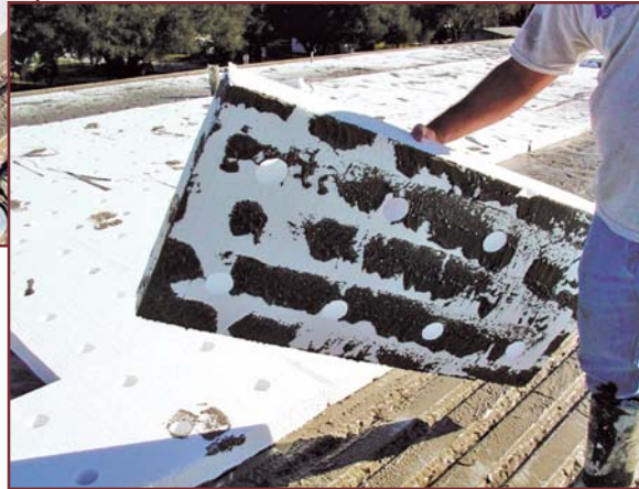
Figures 3A and 3B – Slurry coats with contact at top flutes only.
