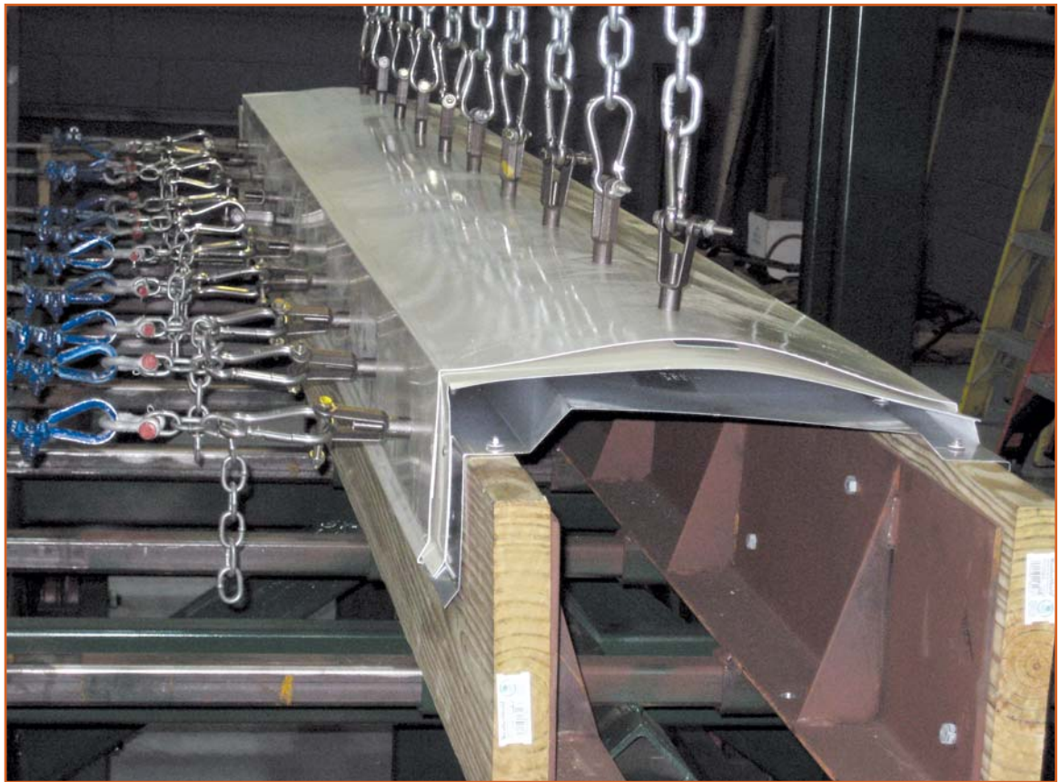
Photo 1 – As part of the ES-1 testing protocol, RE-3 tests upward and outward simultaneous pull of horizontal and vertical flanges of a parapet coping cap. (Courtesy of W.P. Hickman, Arden, NC.)
