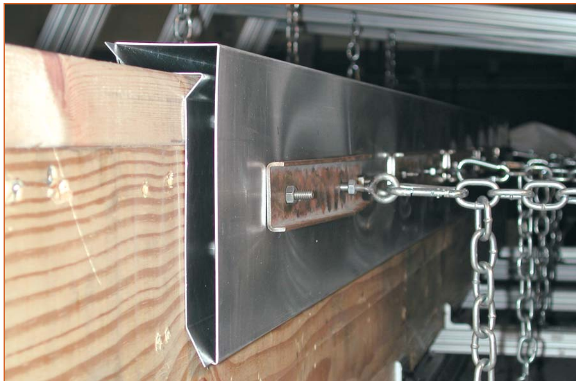
Photo 3 – A metal roof edge system is being tested using a method based on the SPRI/FM 4435/ES-1 standard.
