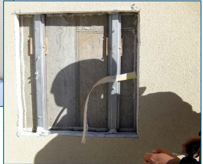
Photo 6 – Test specimen after pull test exposing the metal stud framed wall.
