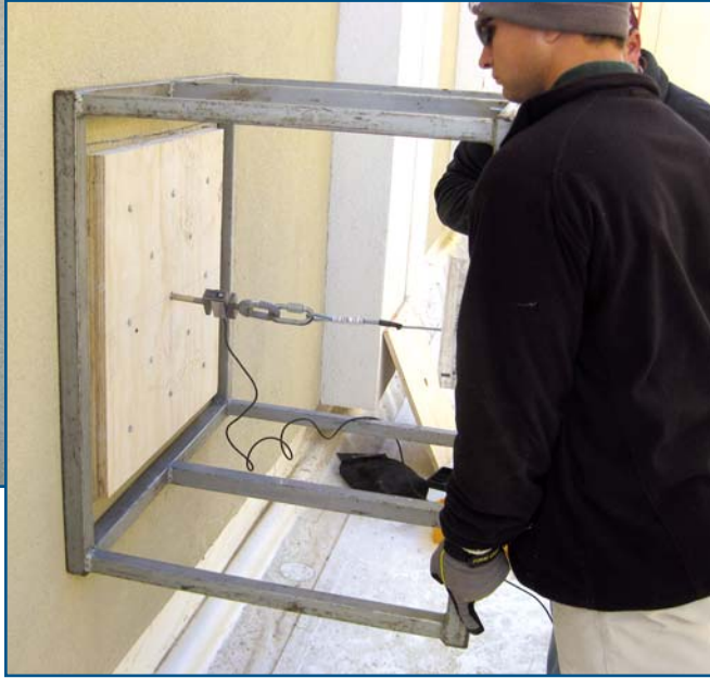
Photo 4 – Pull test frame centered to provide outward pressure on bonded panel.
