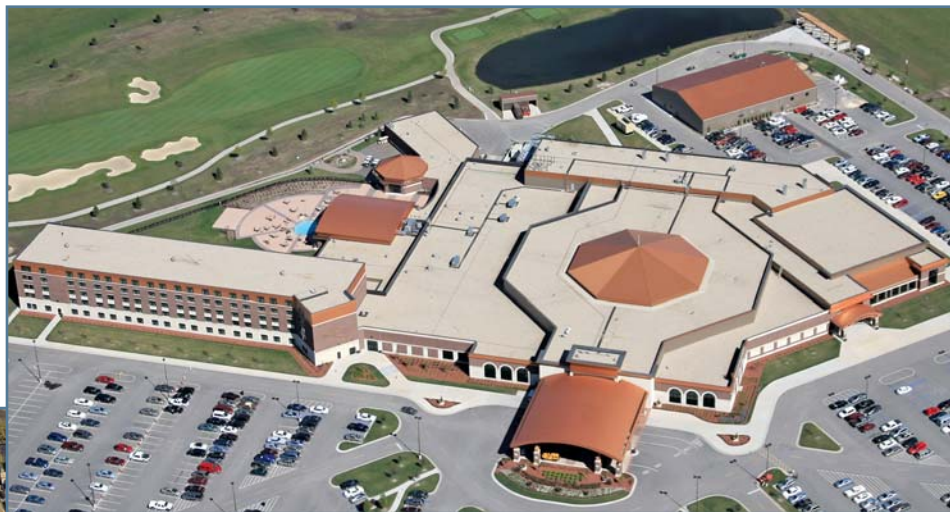
Riverside Casino and Golf Resort in Riverside, IA, chose a light-colored EPDM single ply. (Photo courtesy of Carlisle SynTec, Carlisle, PA.)
