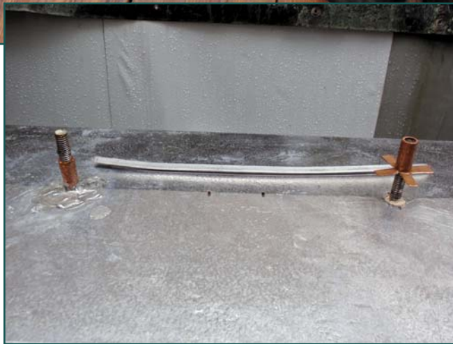
Figure 5B – Close-up of thimbles at dowels.
