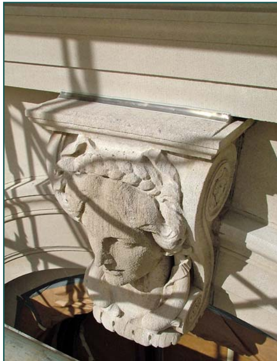
Figure 1 – Small ledge above masonry ornamentation.
