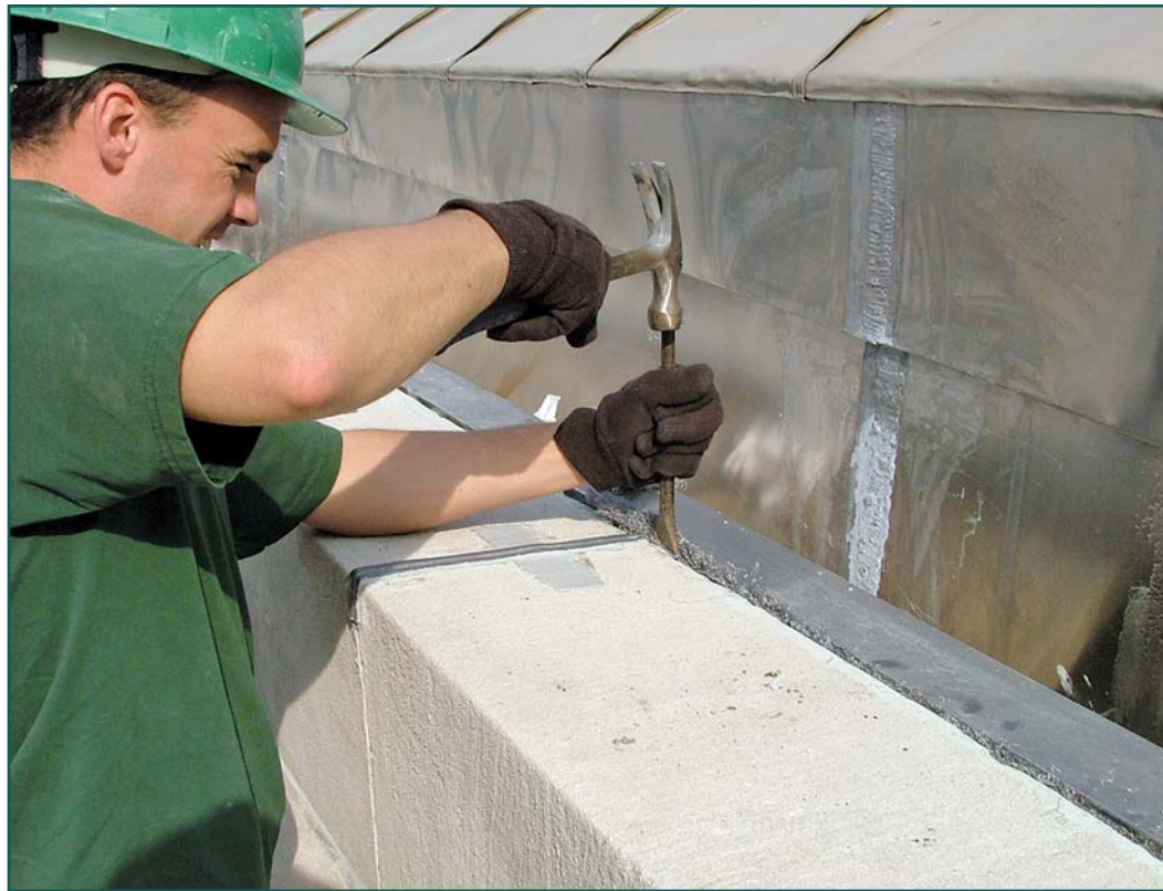
Figure 8 – Lead wool being pounded into place prior to heating.
