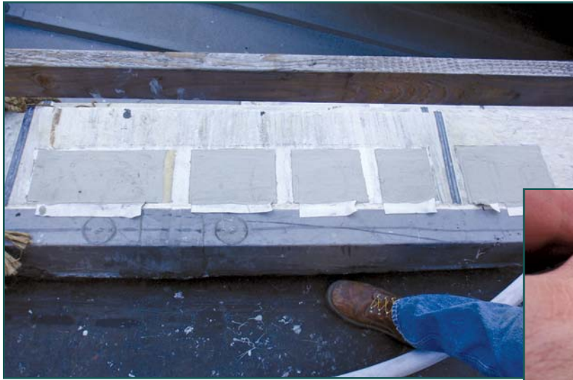
Figure 13 – Mock-ups of different surface preparation for liquid membrane.
