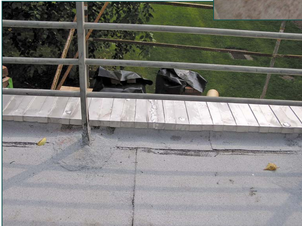
Figure 4 – Three-way interlocking metal under-coping flashing. All seams and fastener heads soldered watertight.
