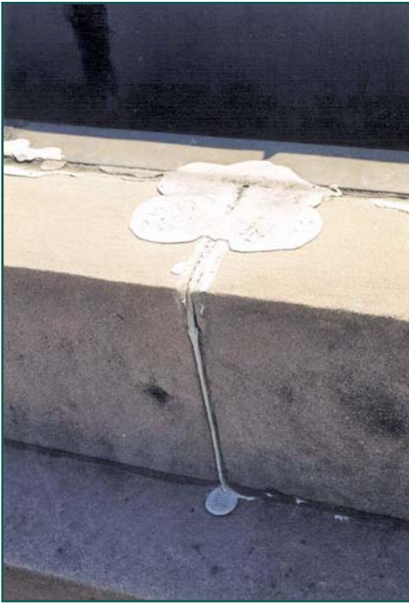
Figure 3 – Self-leveling sealant installed at joints in coping.
