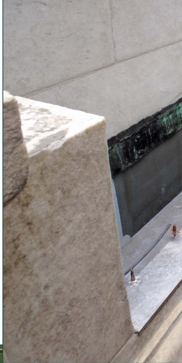
Figure 5A - Metal flashing with dowels.
