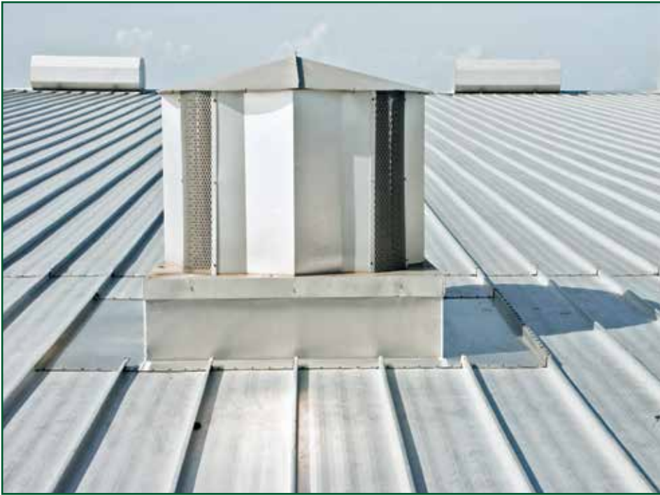
Figure 4 – Preformed structural curbs support weight and seal tightly to the roof.
