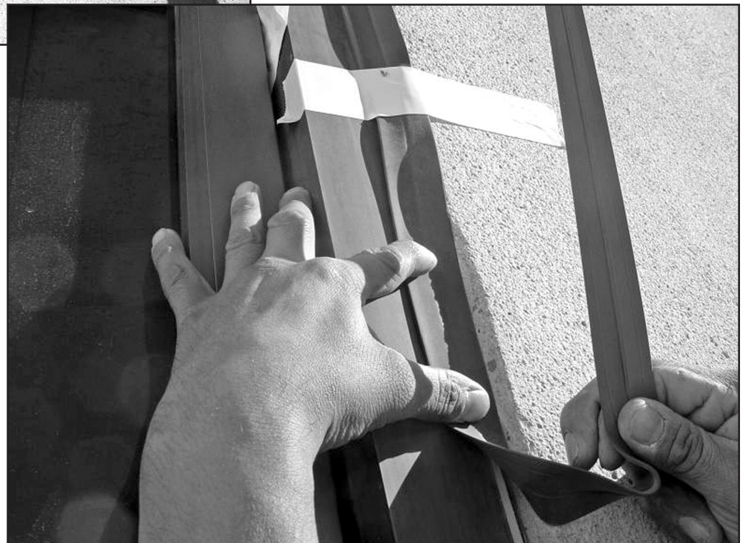
Figure 22 – Precured sealant can handle 200% extension.
