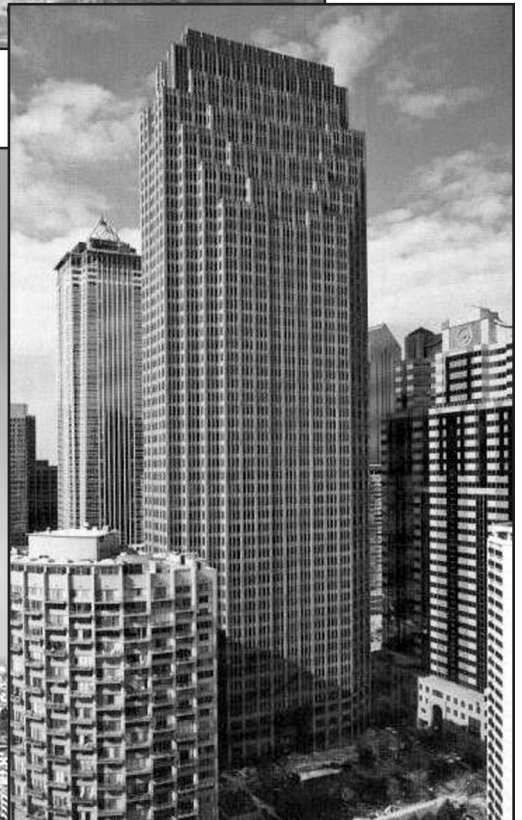
Figure 5 – Bell Atlantic Tower, Philadelphia, PA. Source: Building Design and Construction Magazine.
