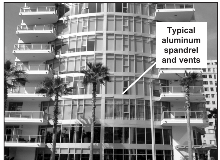
Figure 23 – Segmented window wall.
