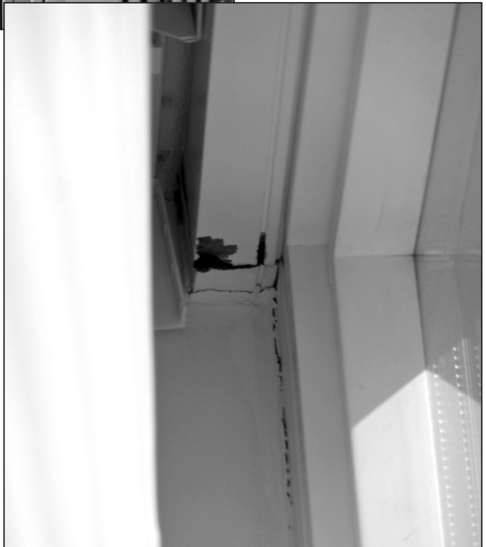
Figure 27 – Interior stains from melting bitumen.
