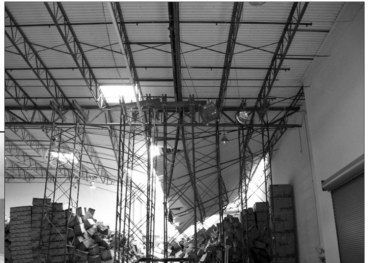
Figure 9—Structural analysis of a building under construction during a storm.
