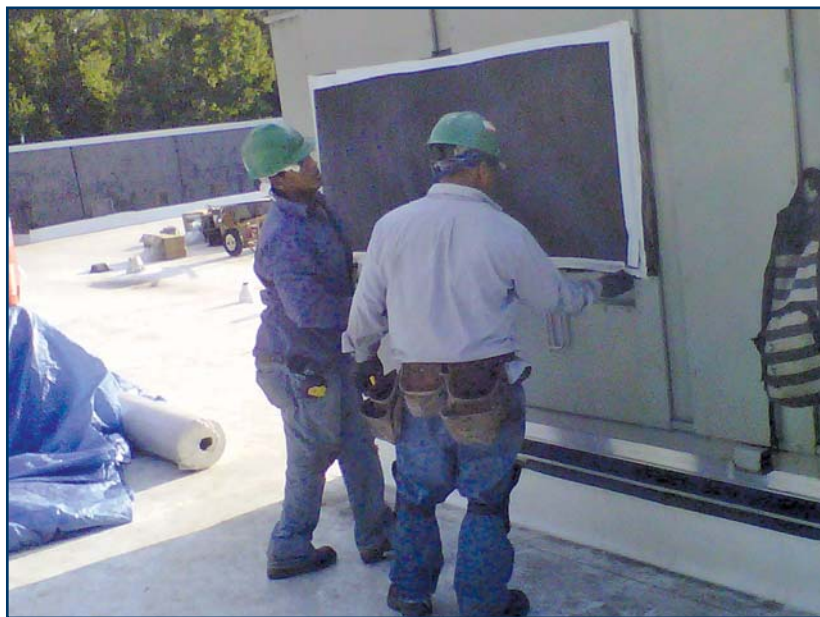
Photo 1 – Intake covering in progress (photo by Dedicated Roof and Hydro-Solutions, LLC).
