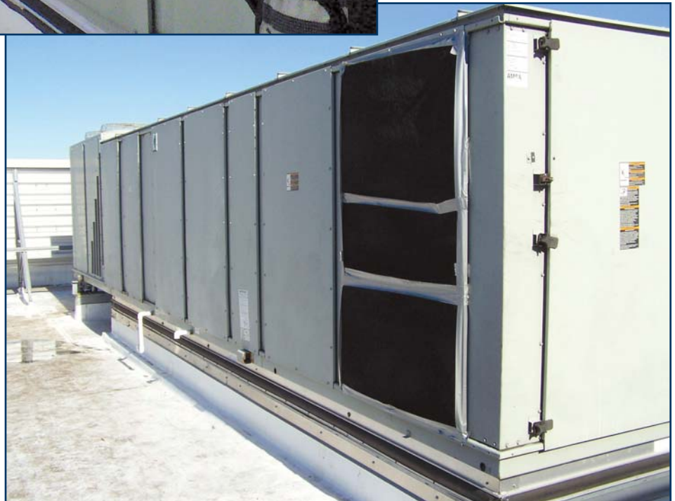
Photo 3 – Example of covered intake (photo by Dedicated Roof and Hydro-Solutions, LLC).
