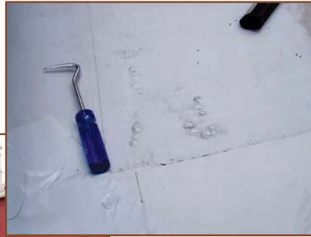
Figure 4 – Blistered membrane caused by extreme heat generated by a highly reflective vertical surface.
