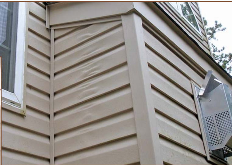
Figure 3 – Distorted vinyl siding after exposure to adjacent highly reflective vertical surface.
