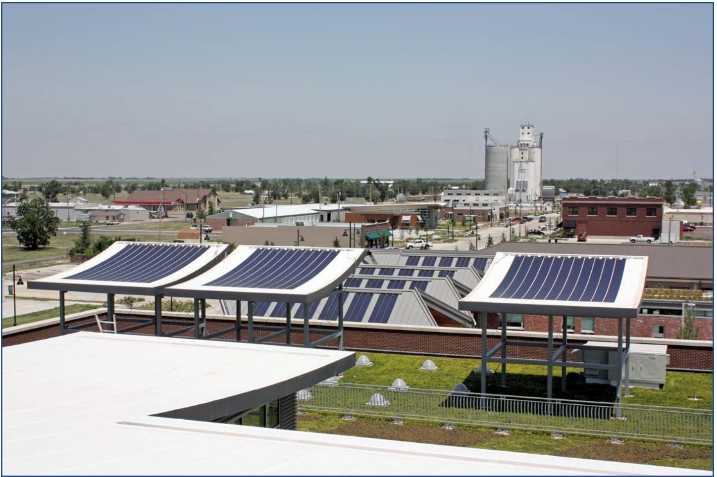
Kiowa County Commons in Greensburg, Kansas, includes high-performance lighting and controls, an enhanced mechanical system, a stormwater runoff collection system, a pair of wind turbines, and water-efficient landscaping, in addition to solar and vegetative roofs. Some of these technologies may also have unintended consequences that must be addressed by the building designer.
