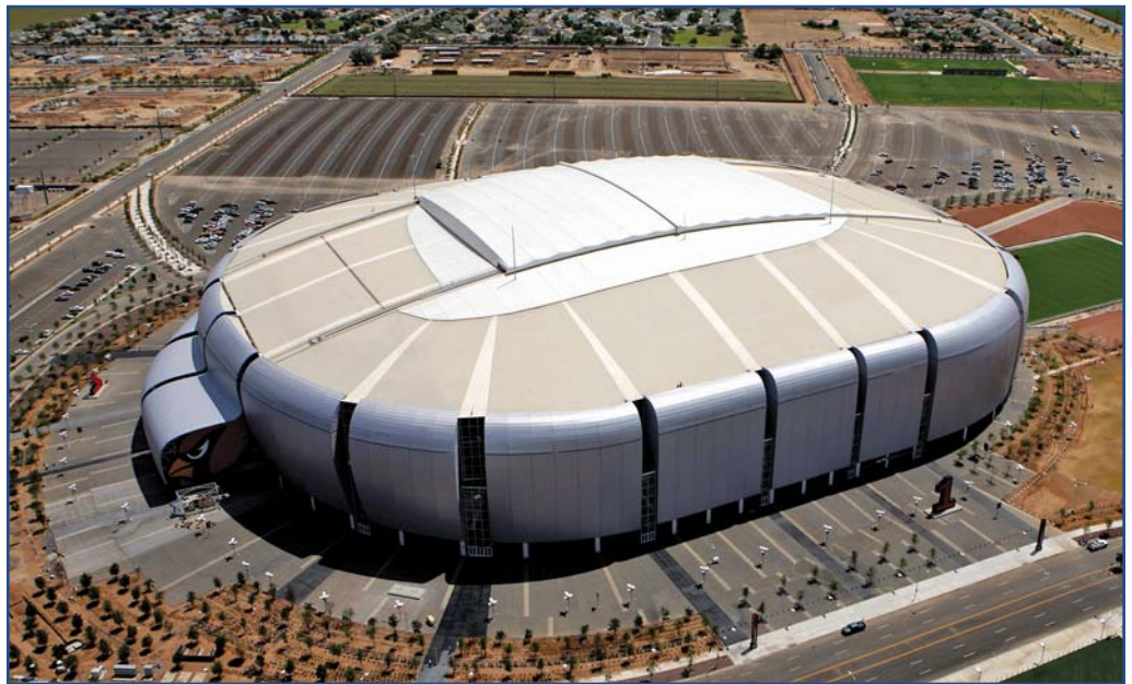
The current generation of TPO membranes has achieved an outstanding performance record in the low-slope roofing market. Shown here is Cardinals Stadium in Phoenix, AZ.
