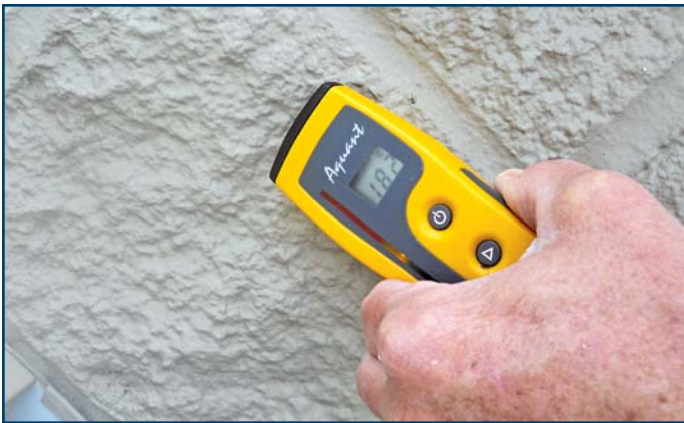
Photo 7 – Instrument used on CMU with coating.
