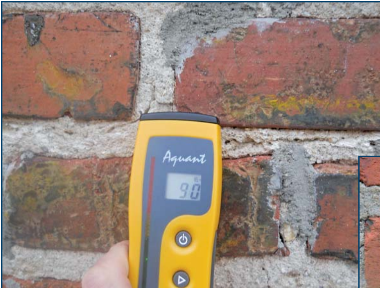
Photo 5 – Low (green) reading on mortar.
