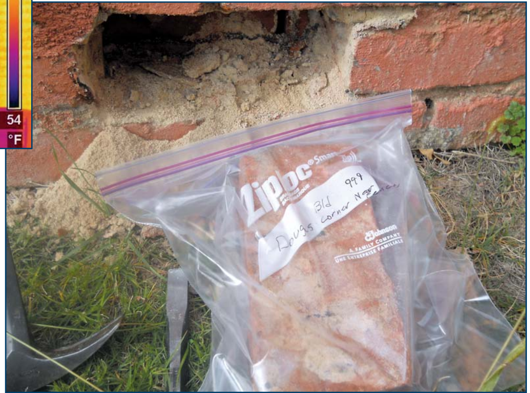
Photo 13 – Brick sample removed to determine percentage of saturation.
