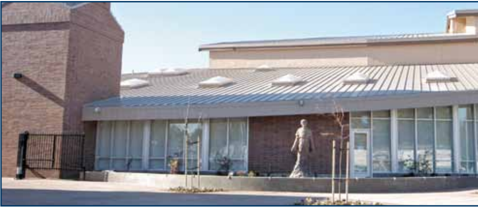
Daylighting is just as applicable in architectural roofing applications as in conventional low-slope applications.
