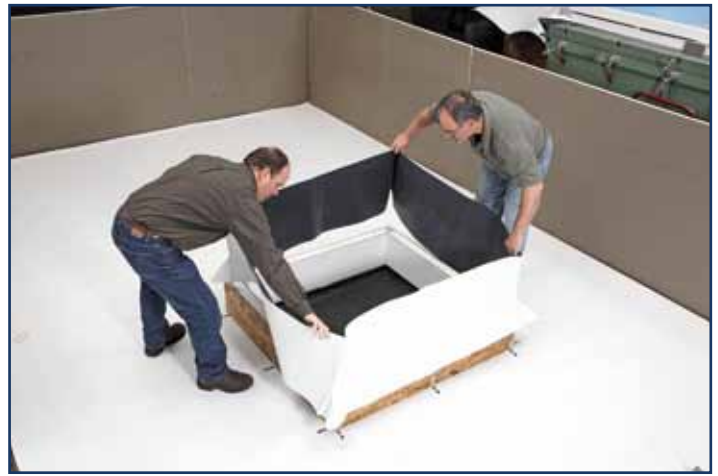
Prefabricated and pressure-sensitive flashings for TPO, PVC, and EPDM single-ply roof systems make it easier for installers to flash in newly installed skylights while increasing overall roof system performance.
