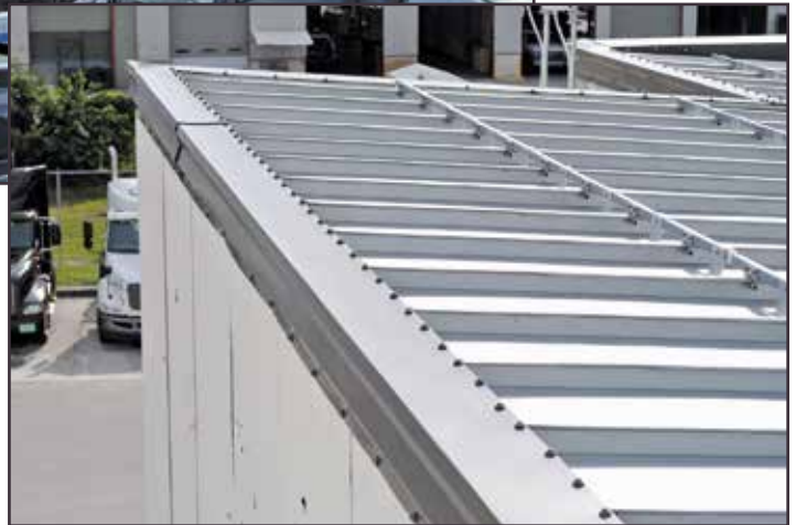
External purlin system on a UPS building in South Florida (photo courtesy of Marc Boulay).
