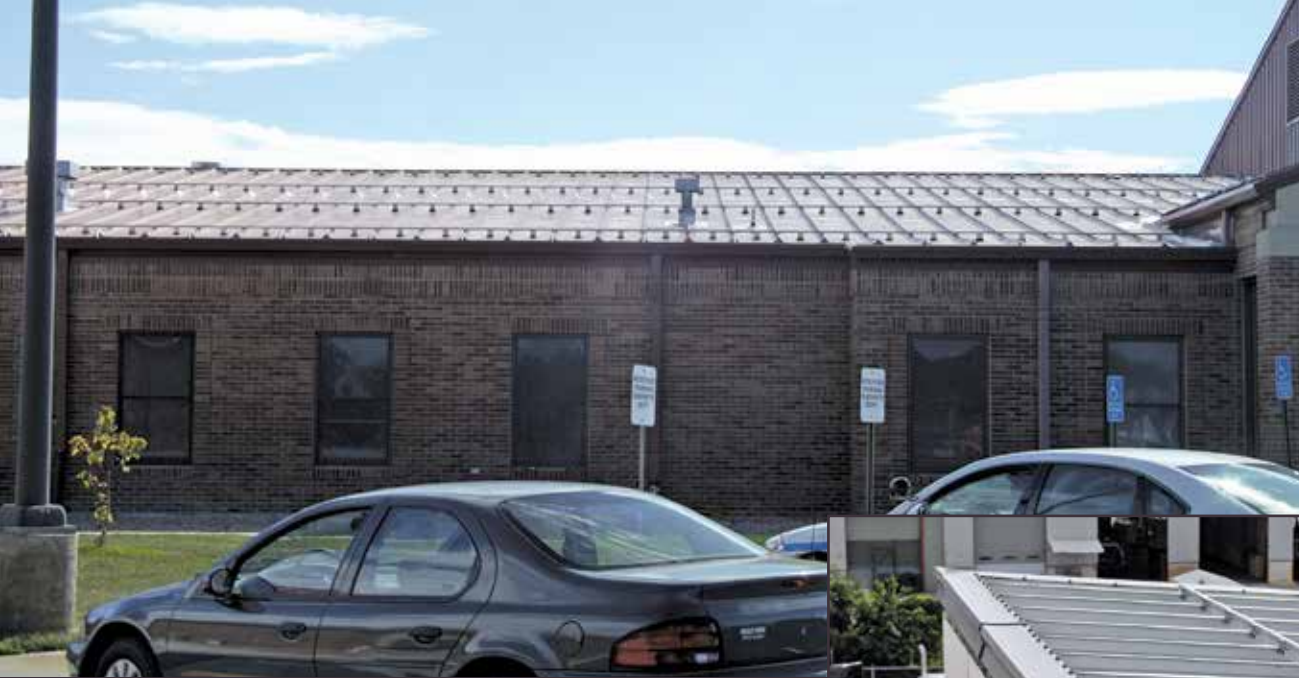
The external purlin system on the Lincoln County Justice Center in Hugo, CO, reduced roof noise due to wind uplift, strengthened the building, and gave snow-retention protection.
