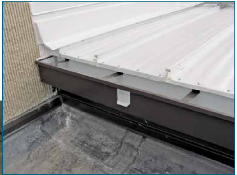
Figure 9 – Vertical-rib panel, fixed at the eave with panel end folded down. Exposed fasteners over the gutter.
