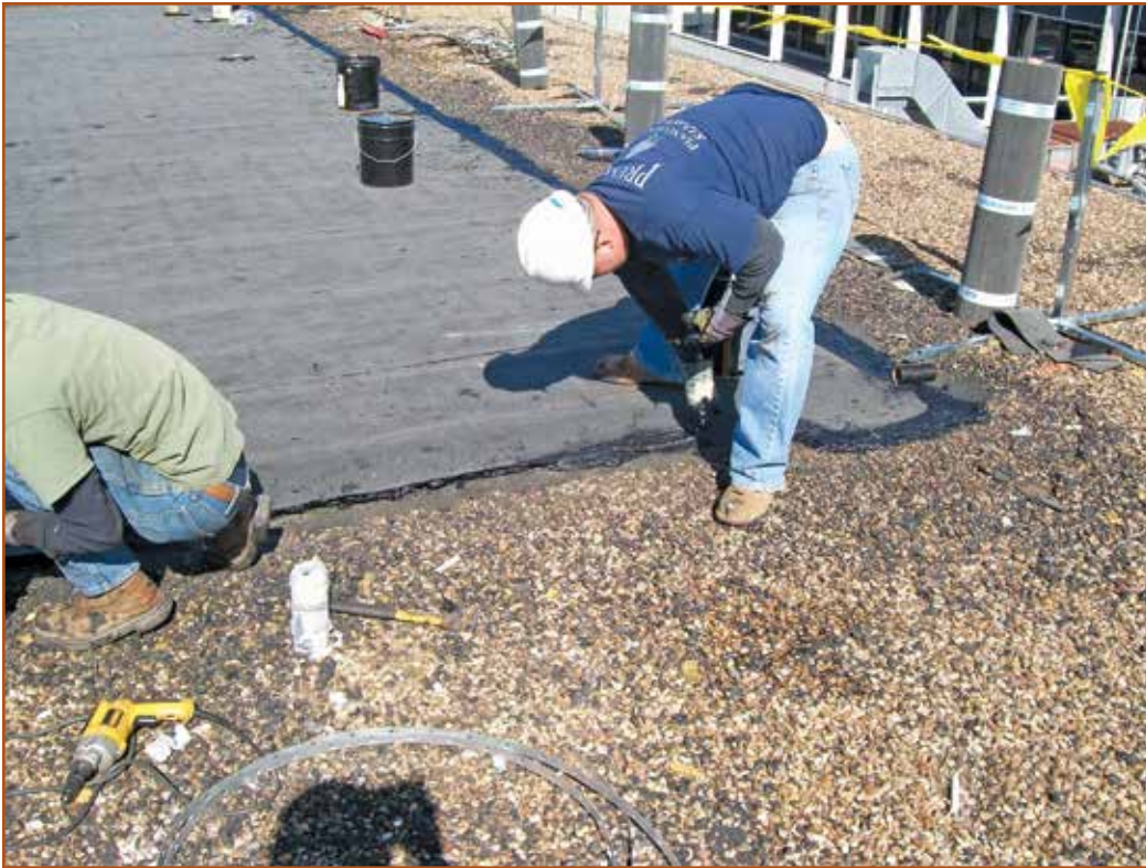
Photo 2 – Plastic cement being applied along edge of tie-in.
