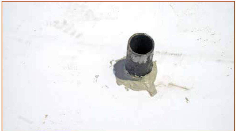
Photo 11 – Sealant applied around penetration in single ply as temporary seal.
