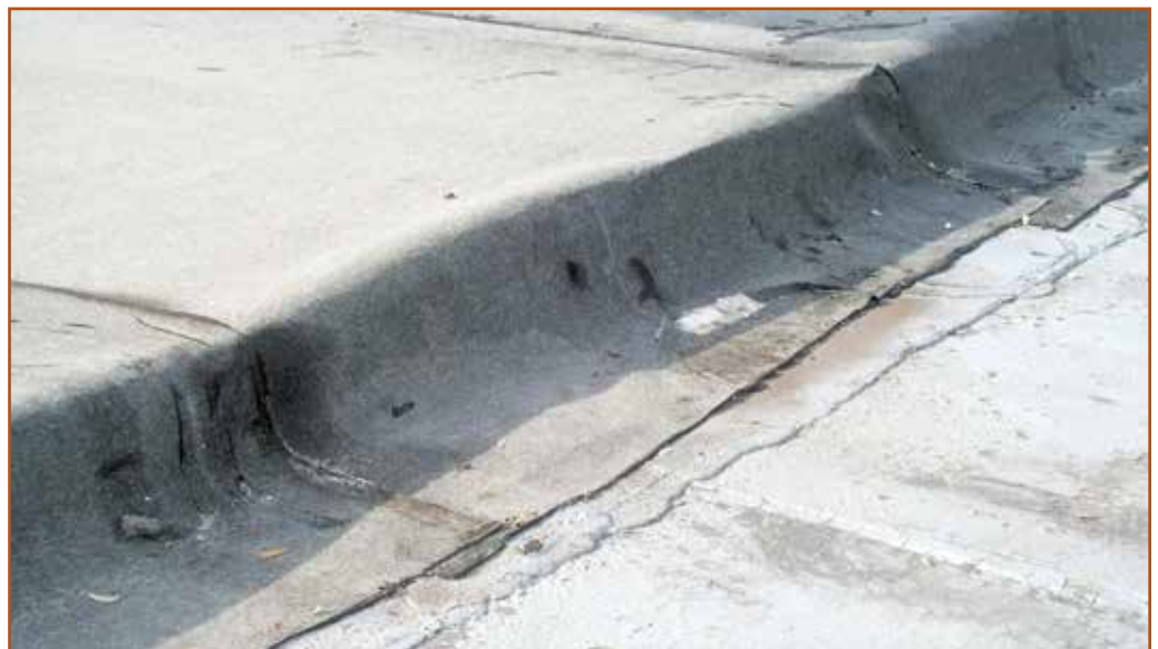
Photo 3 – Tie-in at deck.
