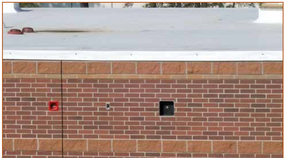
Photo 10 – Trimmed edge of single-ply at perimeter.
