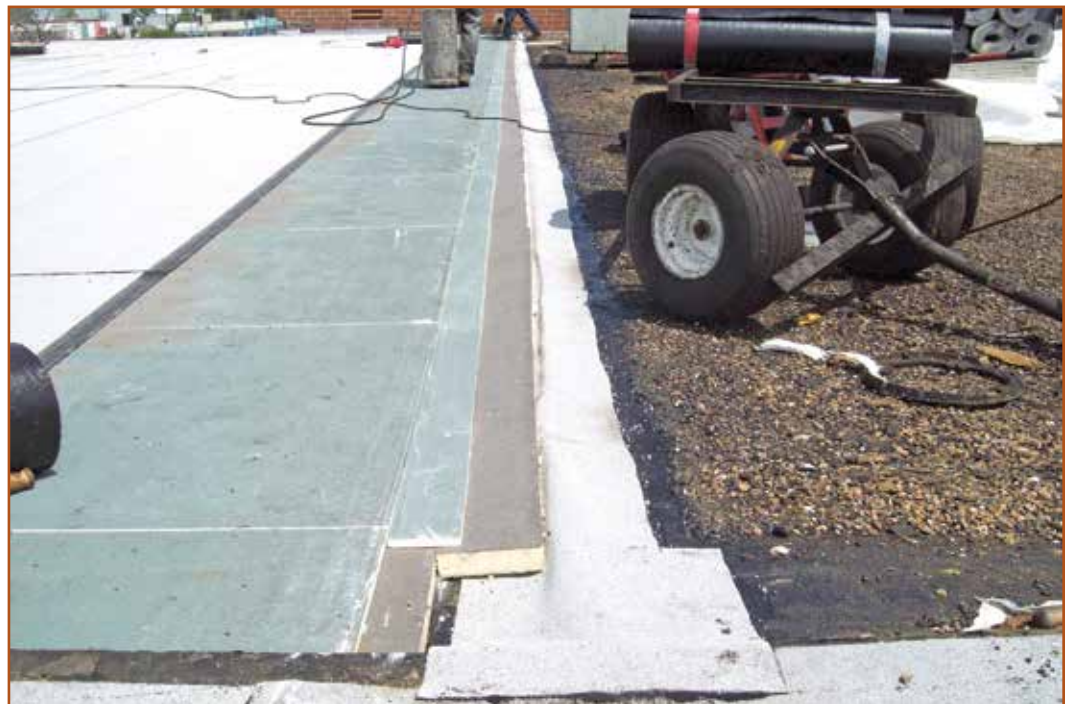
Photo 1 – Tie-in at deck and staggered insulation.
