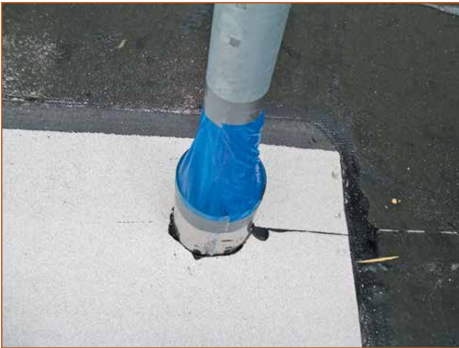
Photo 9 – Plastic sheet and tape applied over top of flashing pan.
