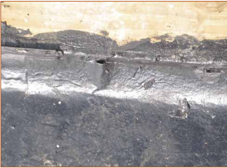
Photo 7 – Open fishmouth at top edge of felts.
