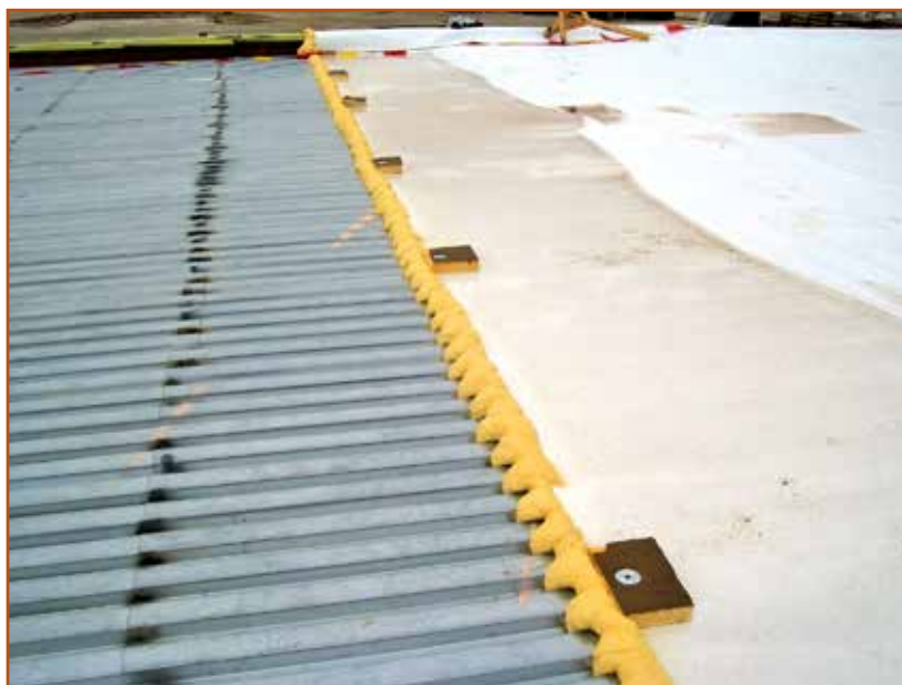
Photo 12 – Spray foam applied along tie-in of single ply on metal deck.
