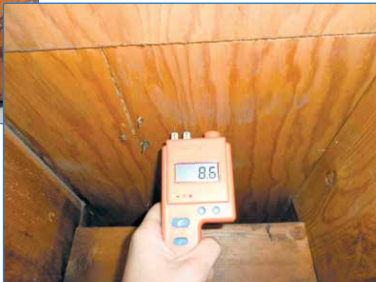
Photo 2 – Adequately ventilated space has moisture content well within acceptable range.
