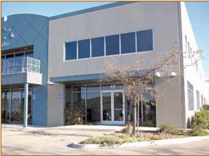
Photo 14 – Phase 2 investigation occurred at Unit 12.
