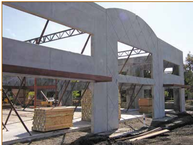
Photo 2 – 2005: Concrete tilt-up panels on “spread footings” surround on-grade concrete slab.
