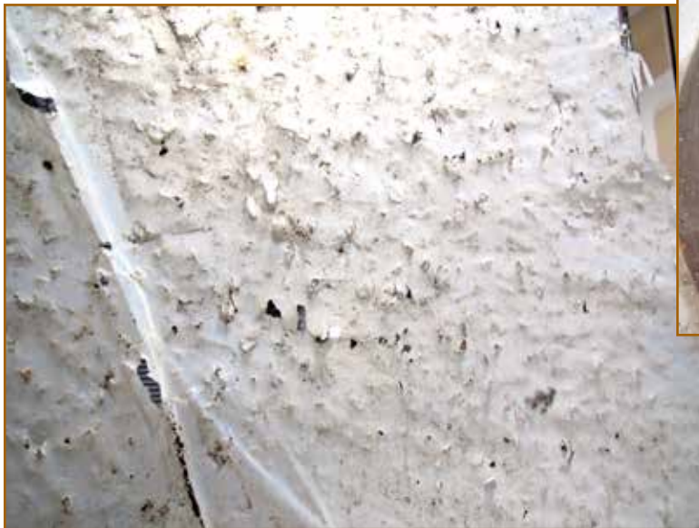
Photo 8 – The polyethylene vapor retarder was found to have numerous punctures.
