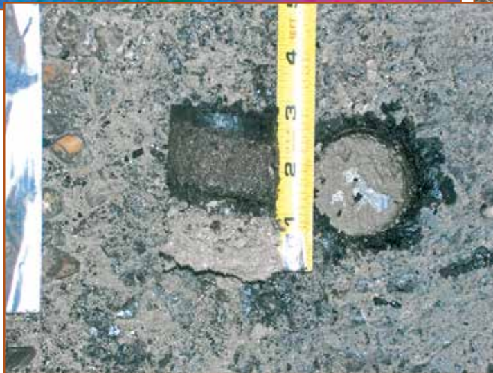
Photo 22 – Core showing wet upper layer of perlite in BUR.
