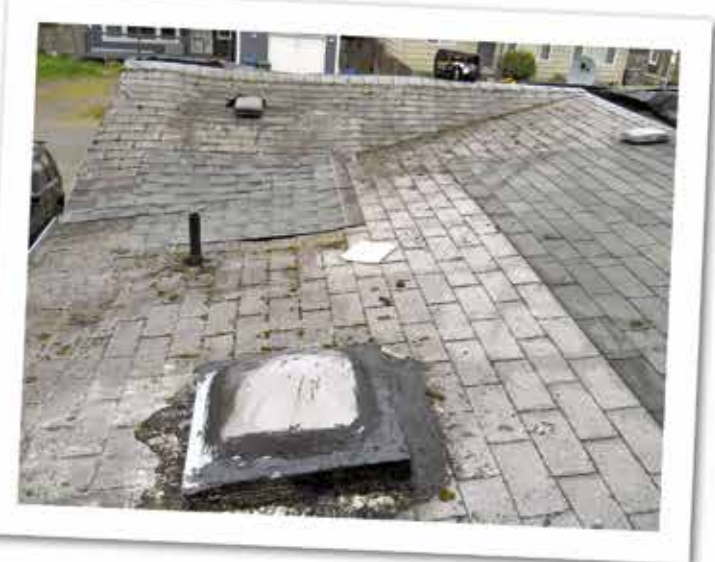
Photo 3 - The exposed roof.
