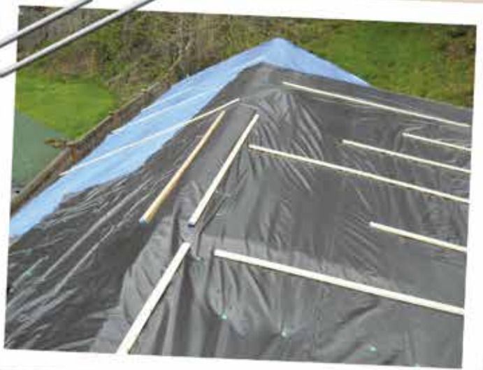
Photo 1 - Visqueen over blue tarp.
