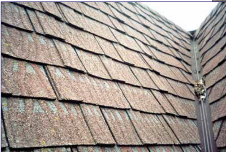
Photo 12 – Shingles on steep-slope section, south end.
