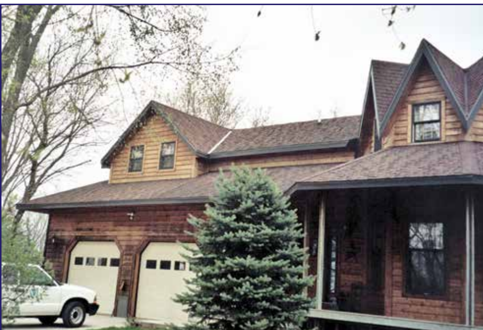
Photo 7 – View of west side (front) and north end of house.
