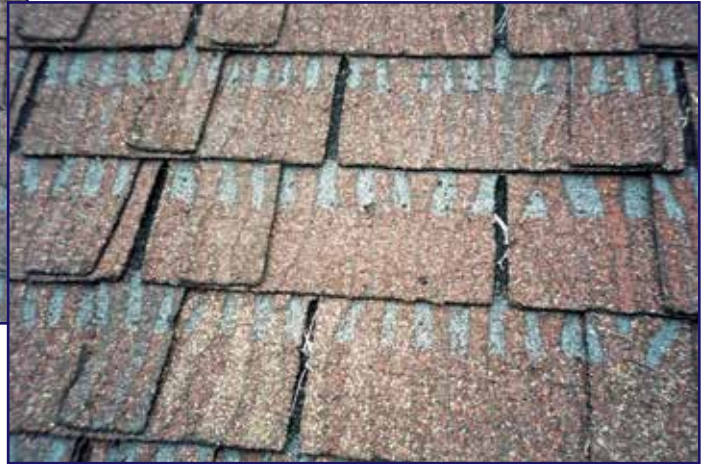
Photo 16 – Close-up of cracking granule surfacing on the south slope of the upper roof north end over the garage.
