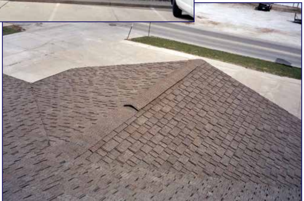
Photo 2 – View of ridge cap and shingles.
