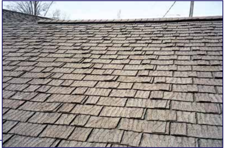
Photo 3 – View of west slope, south end.
