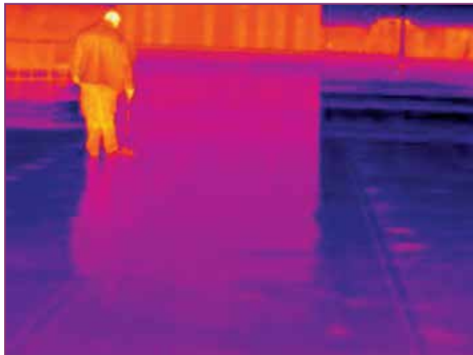
Figure 22 – Reflection due to high angle obscures the roof.
