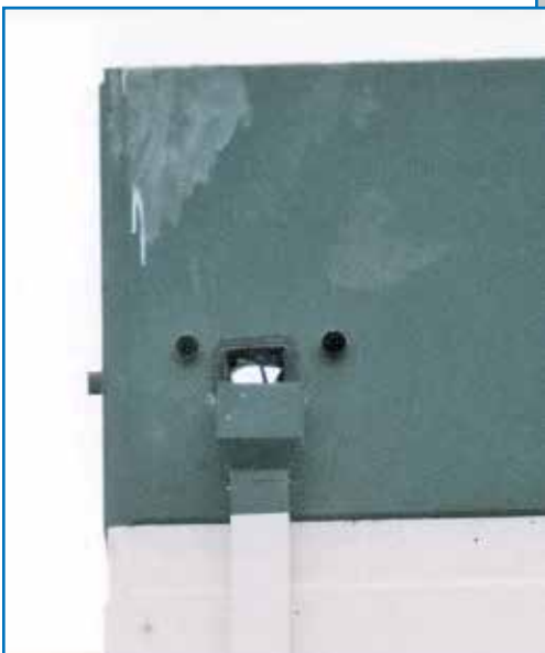
Figure 2 – Roof base flashings covering overflow scupper drains of collapsed roof.
