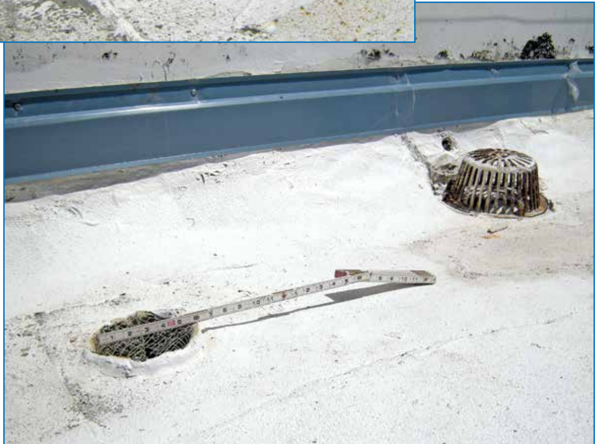
Figure 7 – Five-inch-diameter overflow drain added near drain shown in Figure 5.
