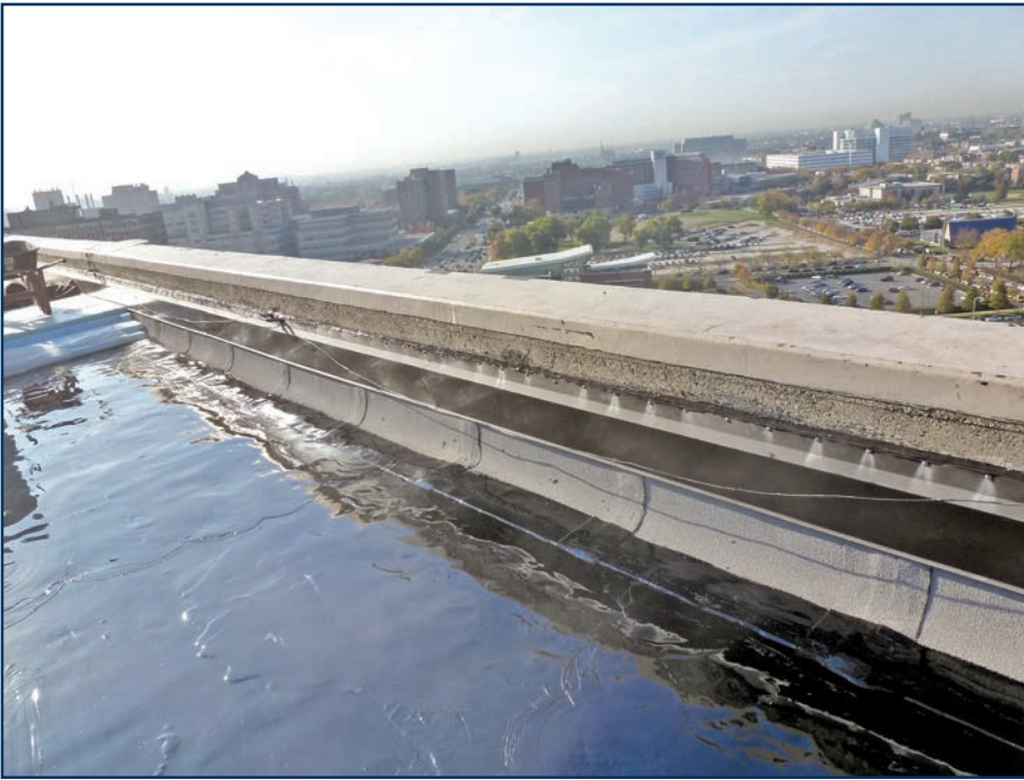
Photo 5 – A PRMA roofing membrane before installation of insulation.
