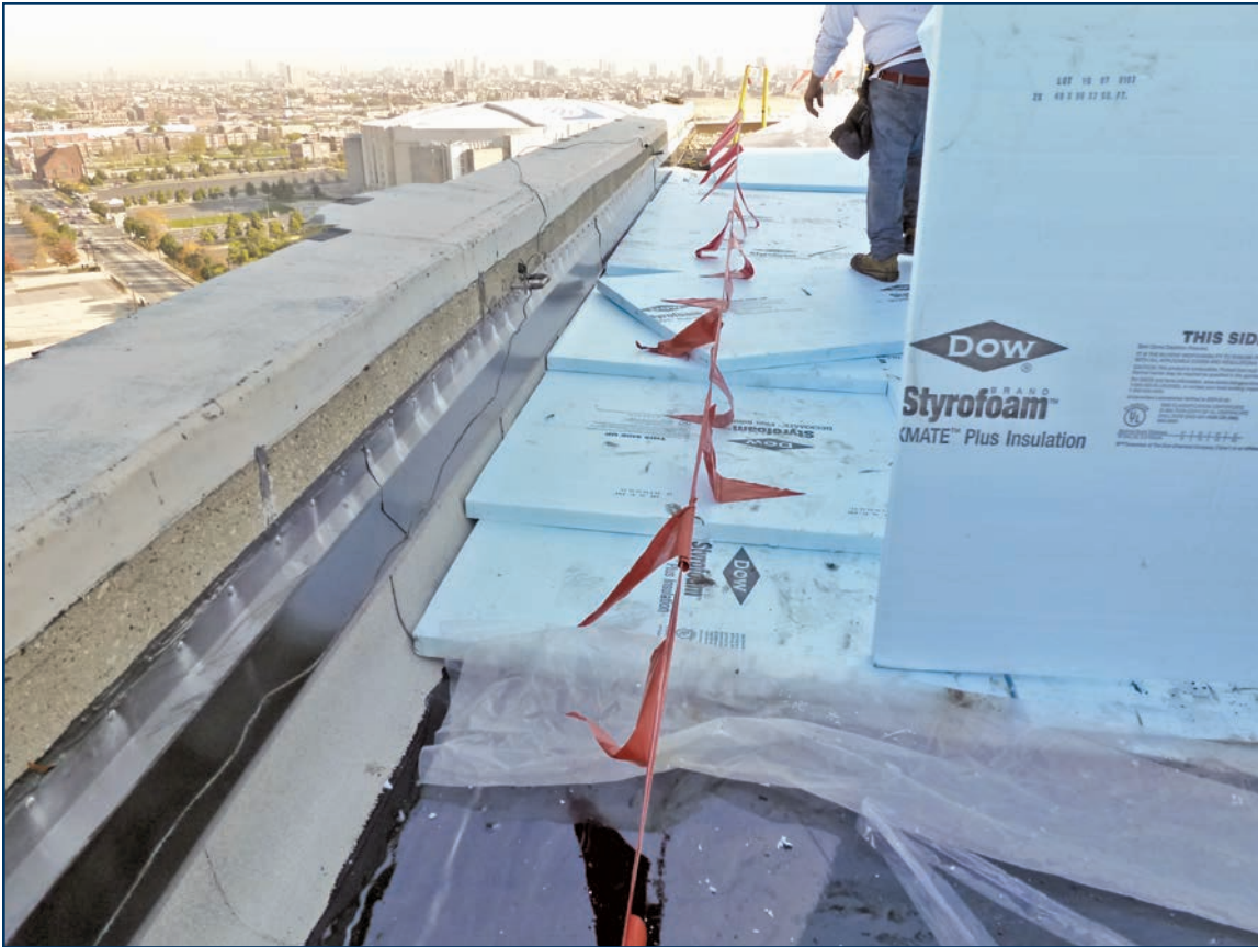
Photo 6 – A PRMA roofing membrane with insulation being installed.
