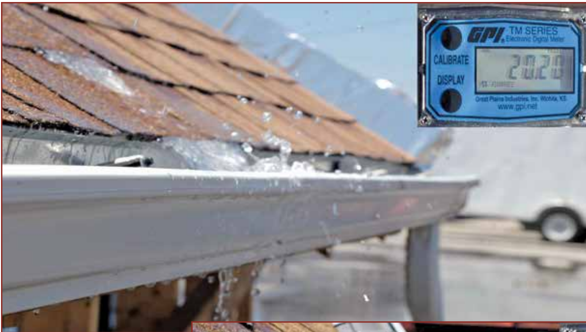
Photo 7 – The flow rate was reduced from 45.0 gpm to 20.2 gpm. Nevertheless, water still overtopped the gutter.
