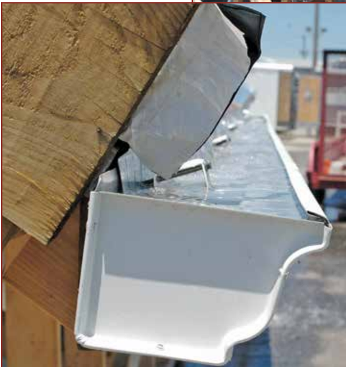
Photo 5 – When the flow rate to the manifold was adjusted to 45.0 gpm, the gutter was completely filled without overflowing. The flow rate per unit length of the gutter was 4.3 gpm/ft.
