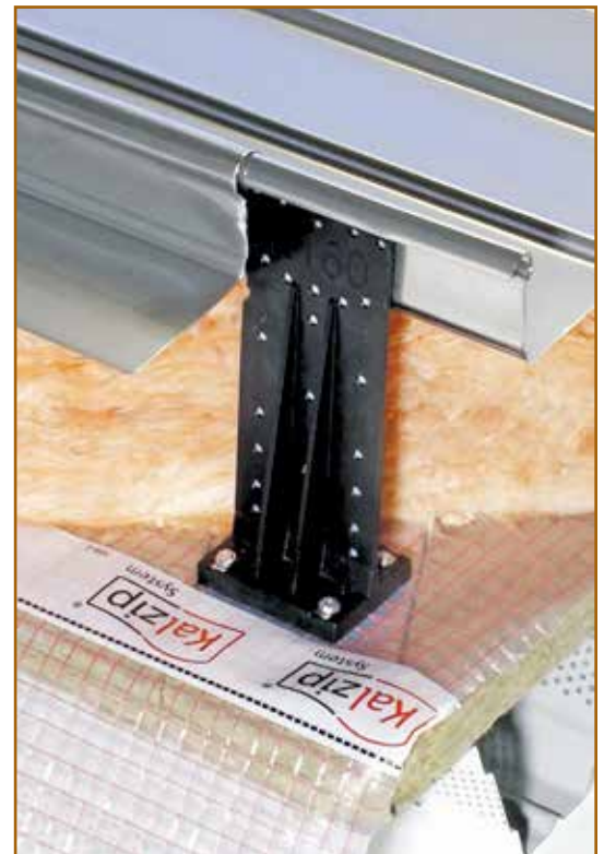
Photo 2 – Typical polyamide clip (halter) detail.
