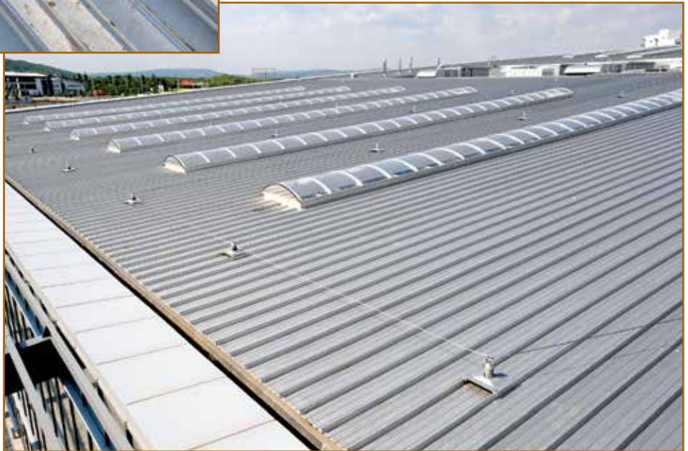
Photo 8 – Tapered aluminum standing seam with welded curb details.
