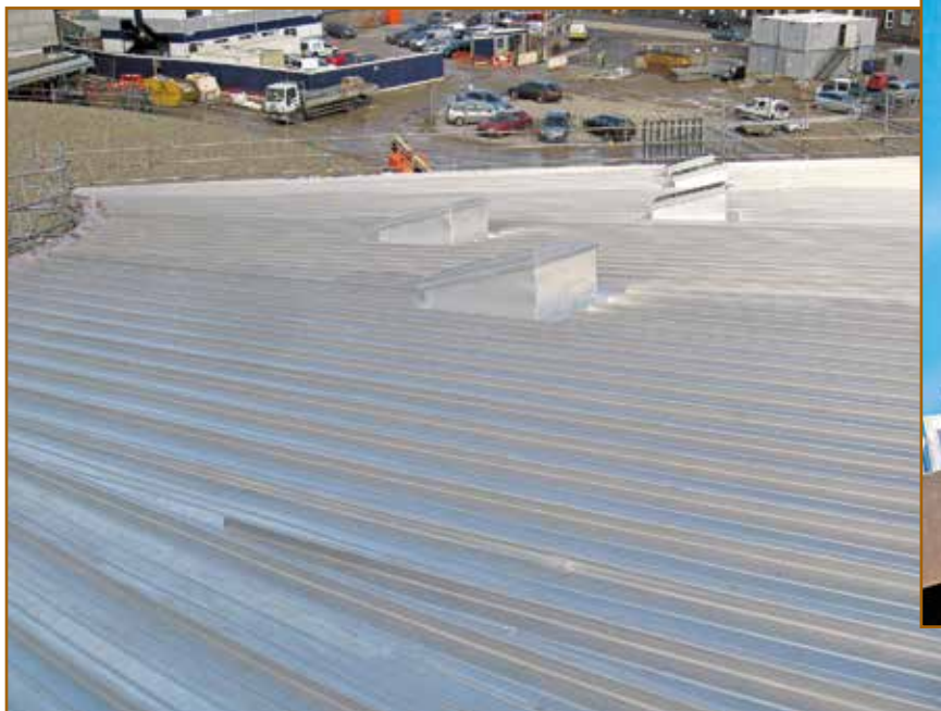
Photo 8 – Tapered aluminum standing seam with welded curb details.
