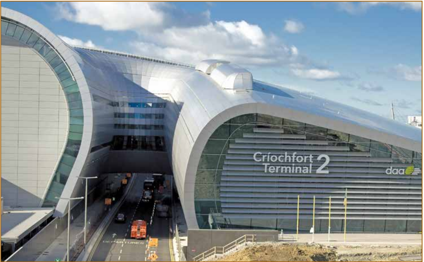
Figure 14 – Composite aluminum panels over curved and low-slope, standing-seam aluminum roof. No penetration of the roof sheet.
