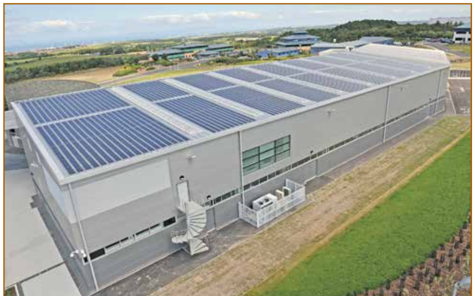
Photo 5 – Low-slope aluminum standing seam with integrated solar panels and skylights.
