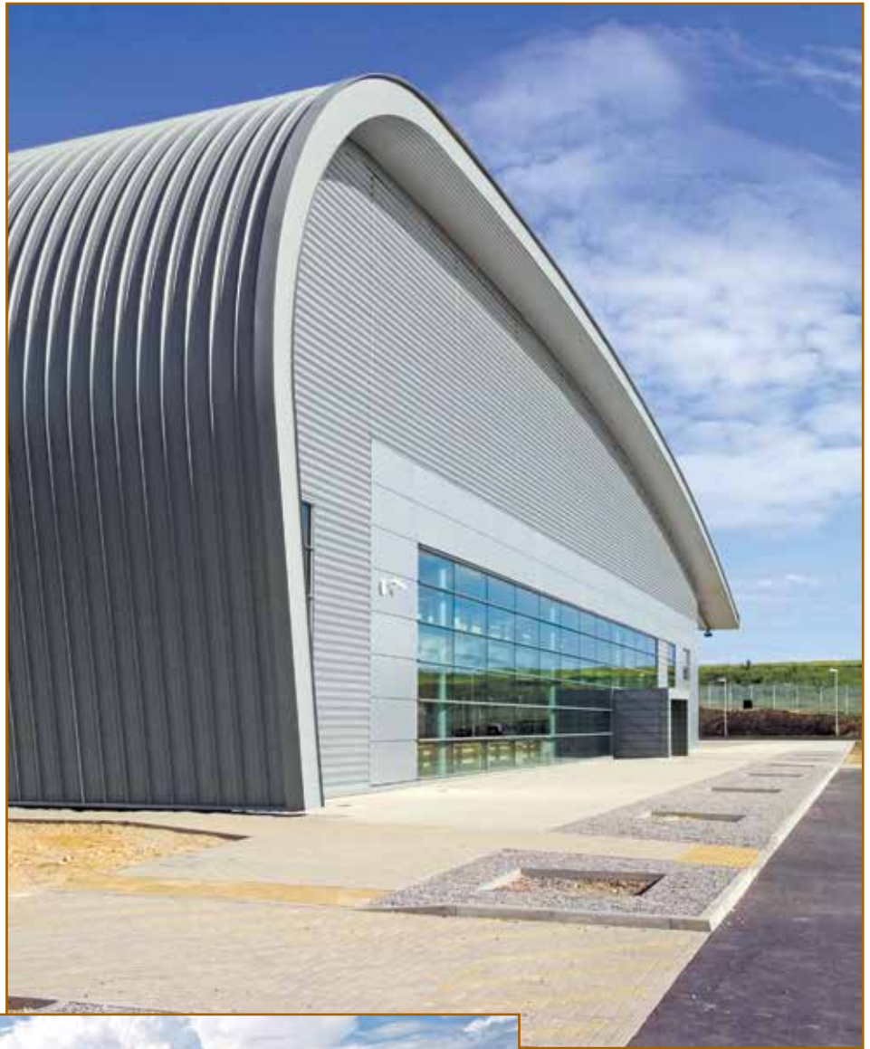
Photo 10 – Typical low-slope aluminum standing seam with curved roof/wall application.
