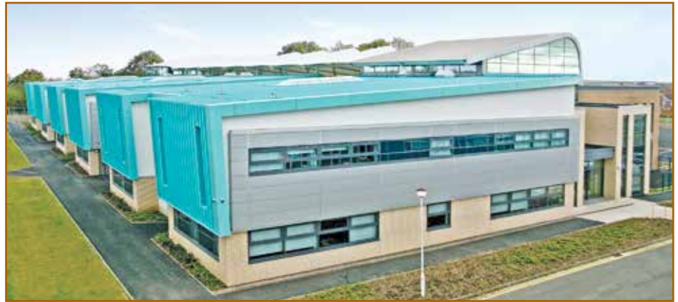
Figure 15 – Low-slope prefinished standing-seam painted and cranked sheets transitioning to wall, plus curved upper roof.
