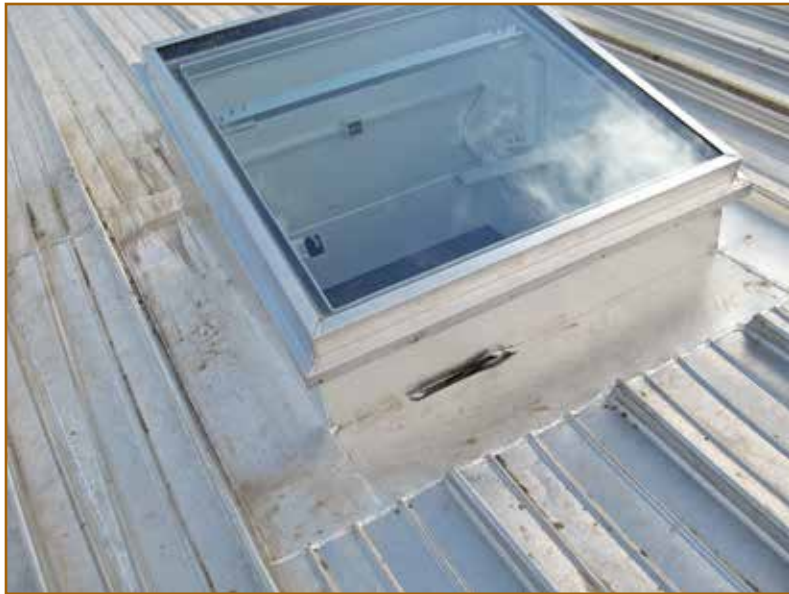
Photo 6 – Small skylight showing welded detailing.
