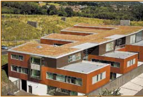
Photo 3 – Low-slope standing-seam aluminum roofing with green roof sections.
