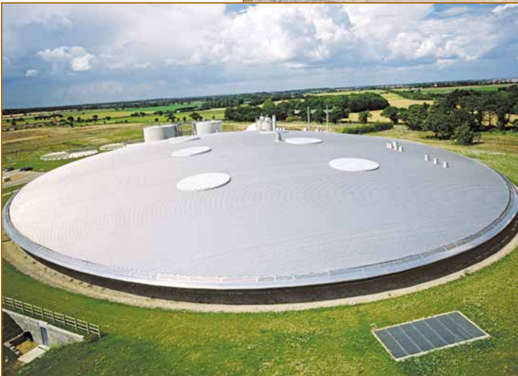
Photo 11 – Low-slope aluminum standing-seam “discus.”
