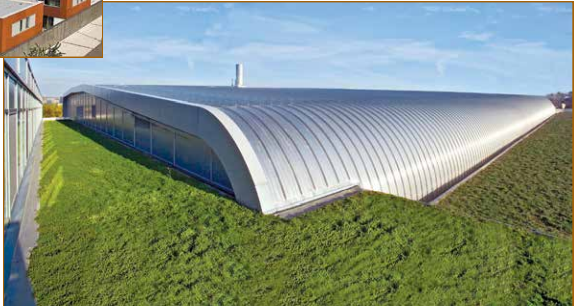
Photo 4 – Arsenal showing vegetated roofing over low-slope standing seam and curved system.
