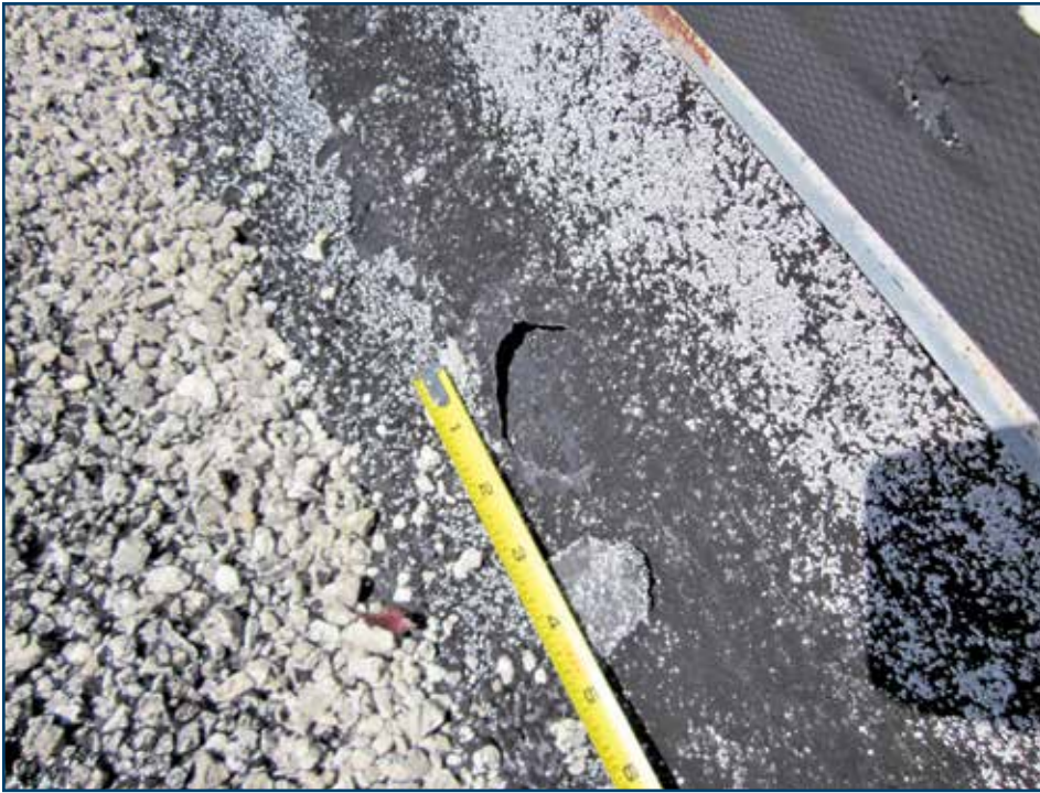
Photo 2 – Unsupported modified-bituminous flashing membrane and resulting hole from hail strike. Note: Gravel-surfaced BUR was otherwise undamaged from the hail.
