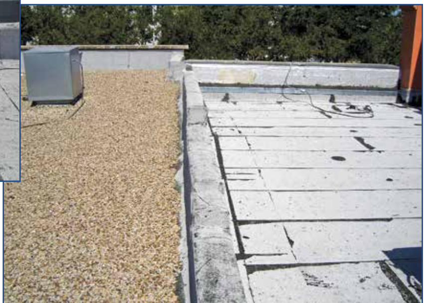
Photo 2 – Aggregate-surfaced BUR and modified-bitumen comparison.
