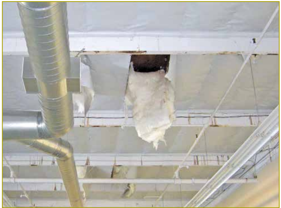
Figure 4 – Water-soaked insulation.
