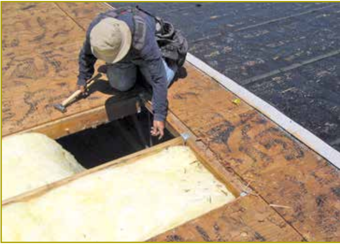
Figure 7 – Roof construction along truss purlins.
