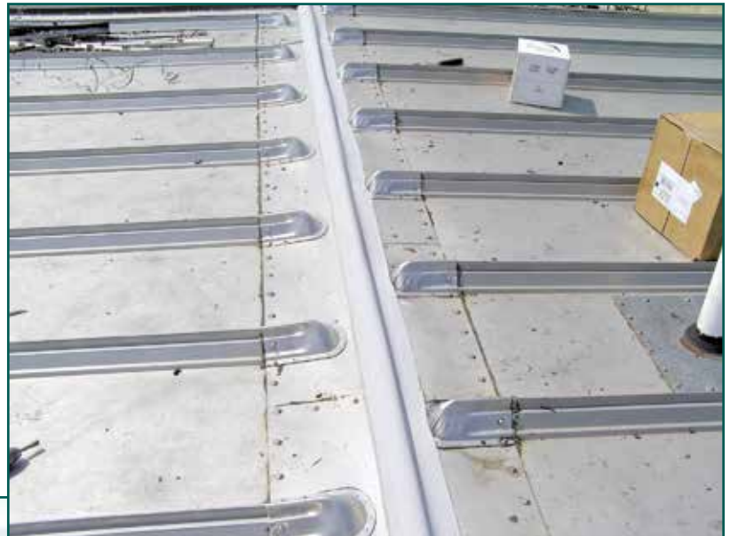
Figure 7 – Metal roof ridge condition sealed using precured silicone sealant.
