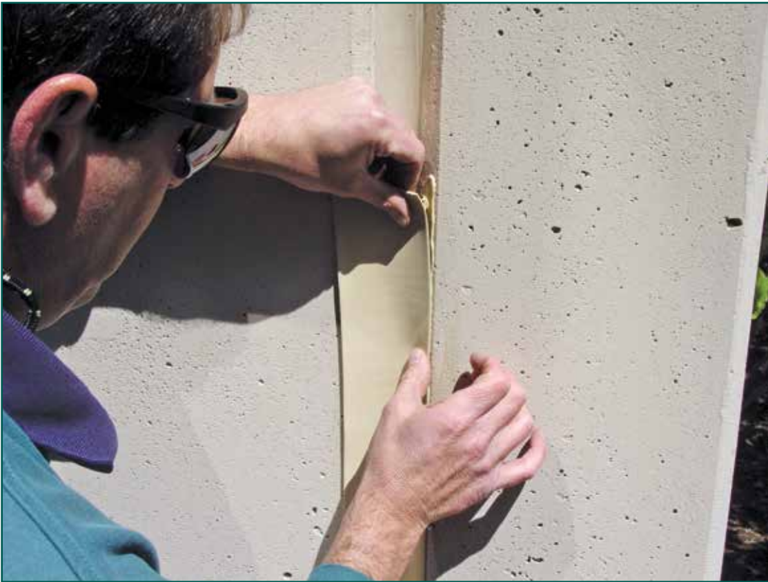
Figure 3 – Pre-cured silicone sealant repair joint installation.
