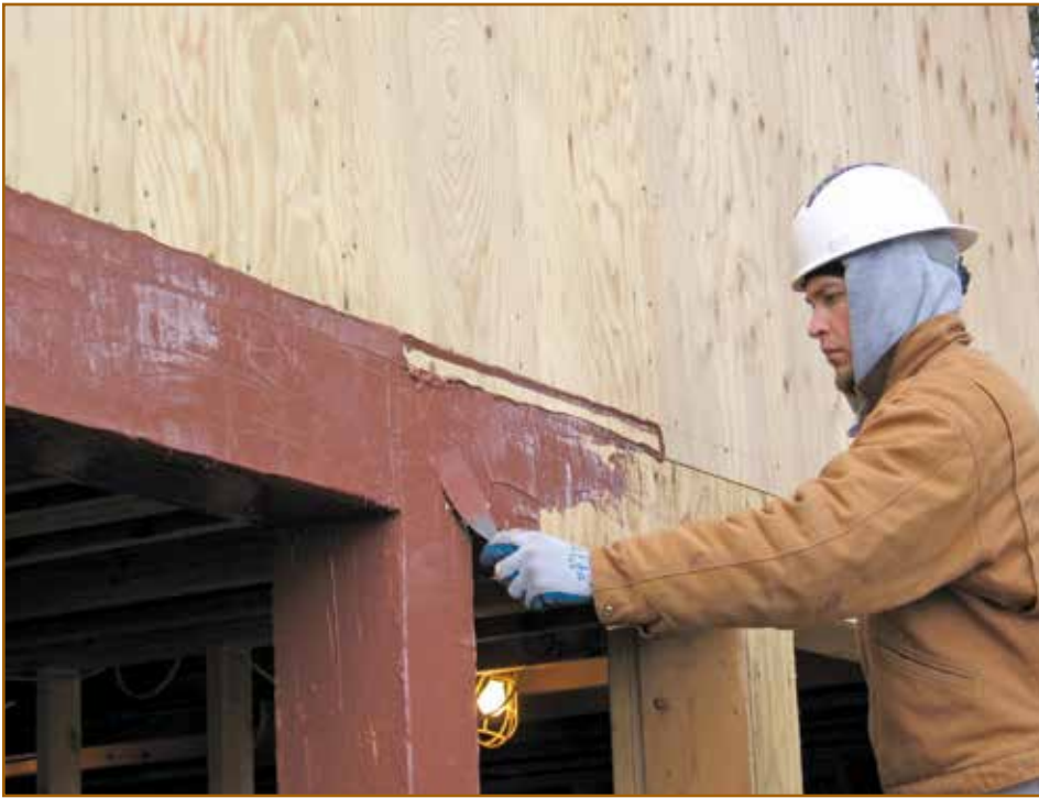
Figure 3 – An applicator demonstrates the relative simplicity of waterproofing a rough opening with the STPE-based flashing system. Photo, courtesy BEI, LLC.
