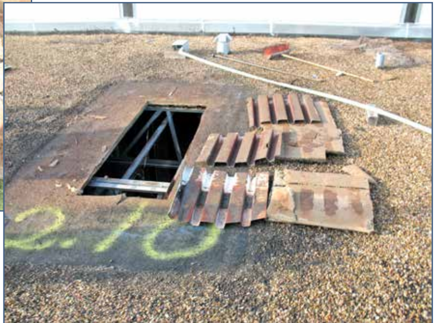
Figure 2 – Metal deck samples with corresponding section of fiberboard insulation.
