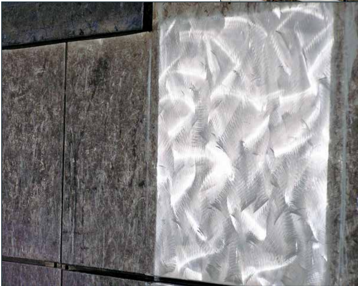
A marked contrast is apparent after cleaning of a stainless steel building in Denver.
