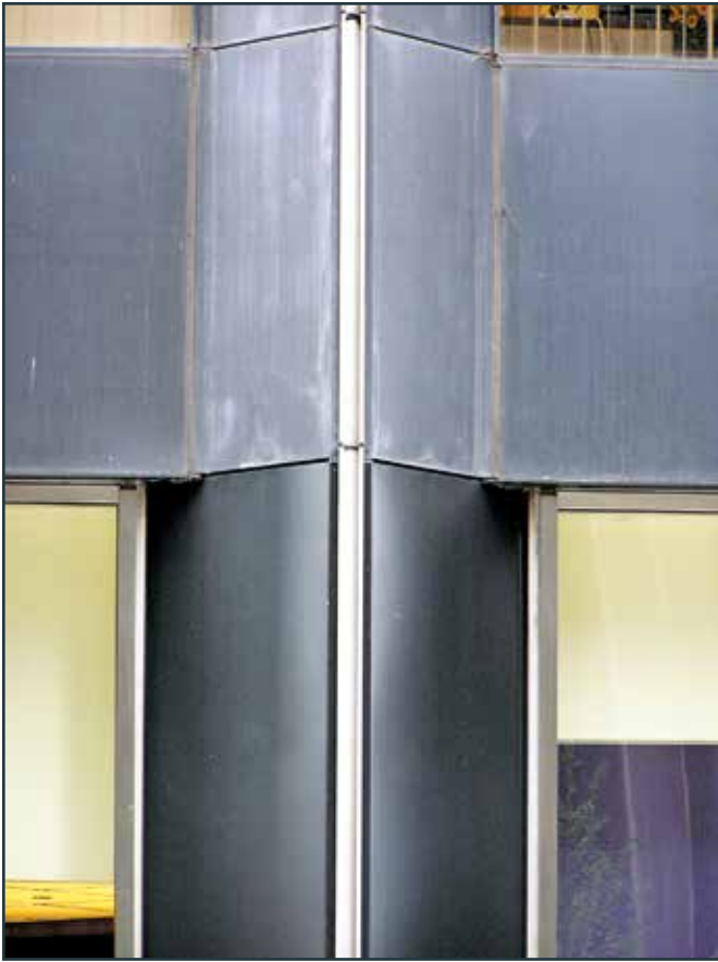
Note contrast before (top) and after (bottom) restoration of black anodized aluminum.
