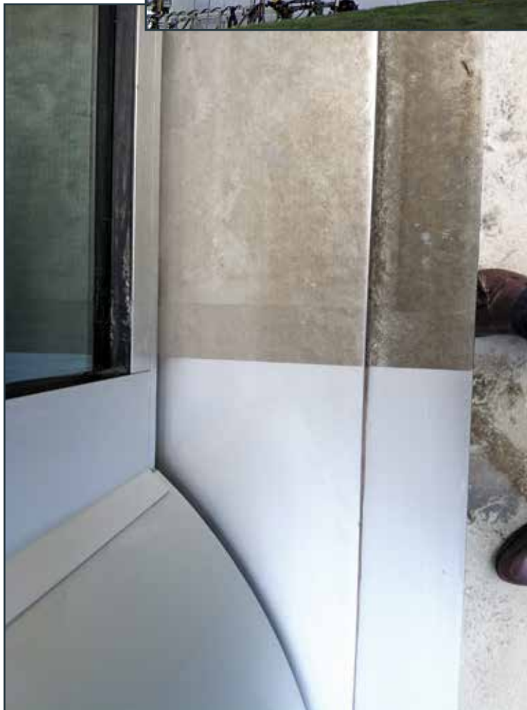
Close-up of painted aluminum cleaning contrast.
