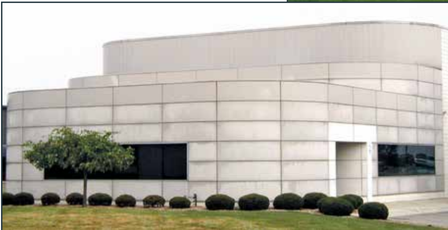
Painted composite panel restoration before.
