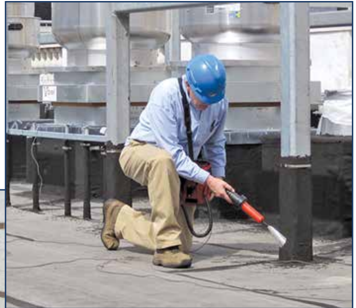
Figure 6 – High-voltage testing is excellent for vertical surfaces and congested areas.
