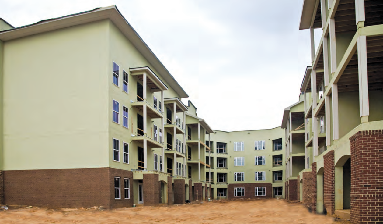
Figure 2 – Installed fluid-applied barrier.
