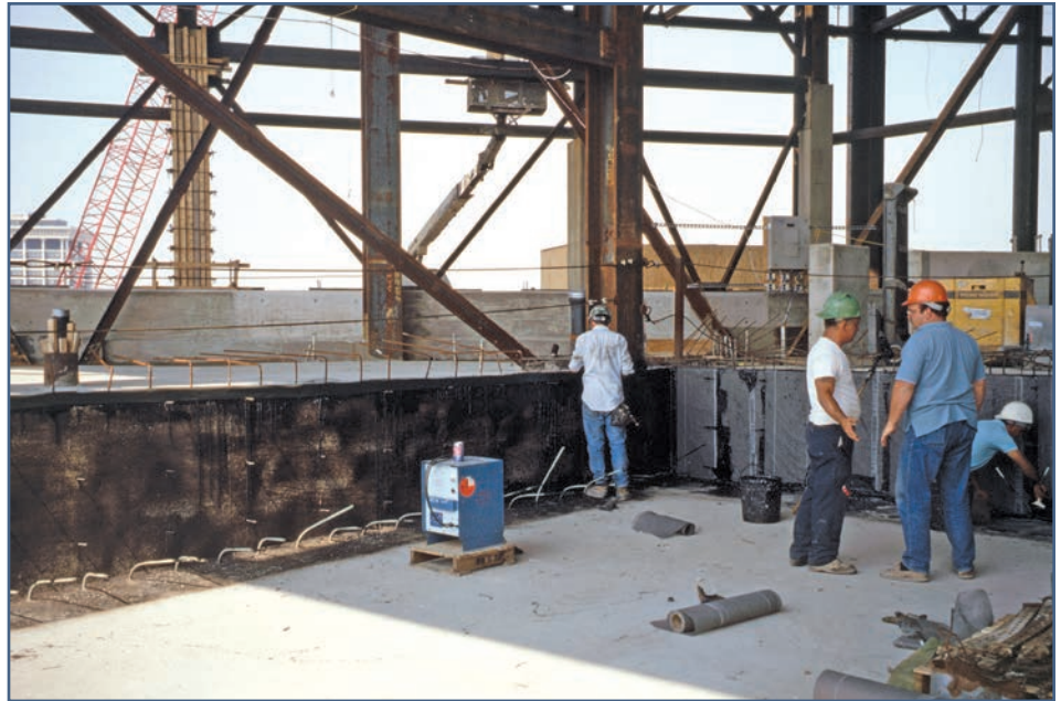
Photo 7 – Installing rubberized asphalt wall flashings (McCormick Convention Center, Chicago).
