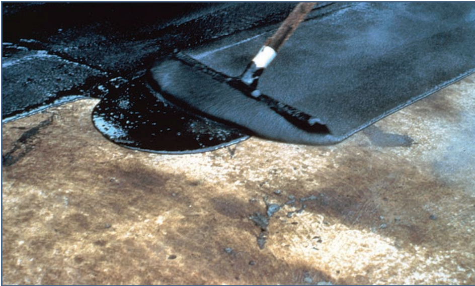
Photo 2 – Fluid material being spread with a squeegee.
