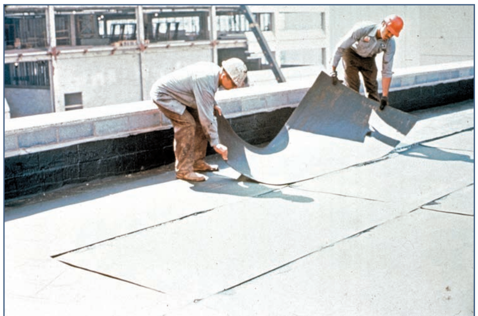
Photo 6 – Installing protection course.
