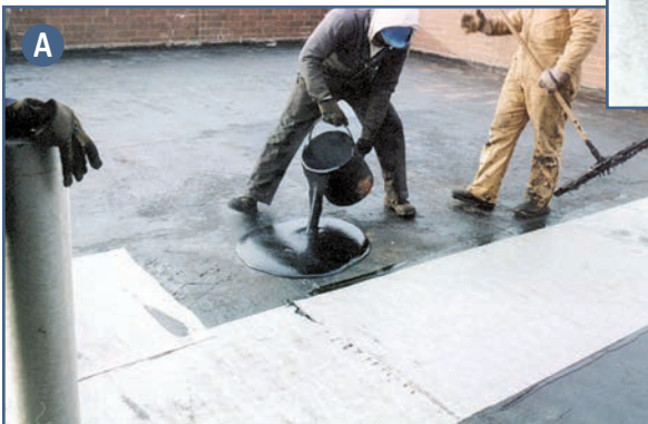
Photos 3A-3C — Installing and overcoating polyester reinforcement.
