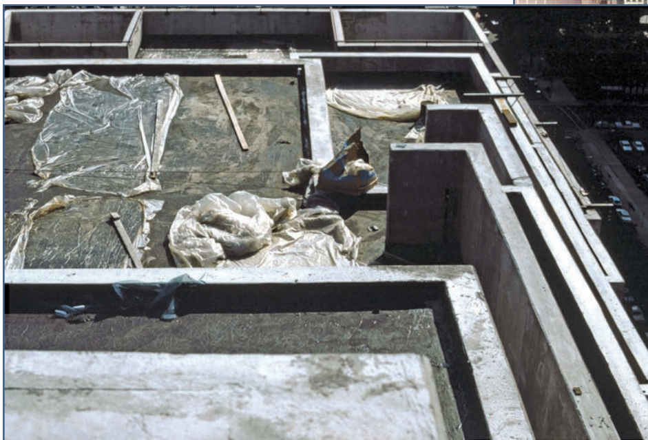
Photos 11A-11B – Waterproofing a high-rise swimming pool and plaza.
