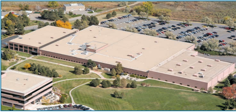
Photo 2 – This built-up roof is both attractive and reflective.
