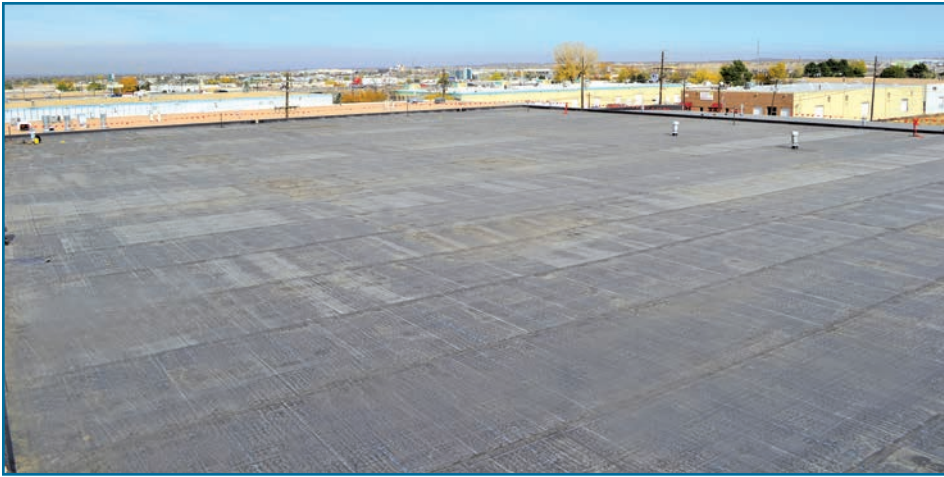
Photo 5 – Nongravel BUR surfacing options include aggregate, mineral surface cap sheet, or a smooth, surface-coated membrane. After many years of exposure to the elements, all of these surfacing materials may need some attention due to possible aging and weathering of the BUR surface.
