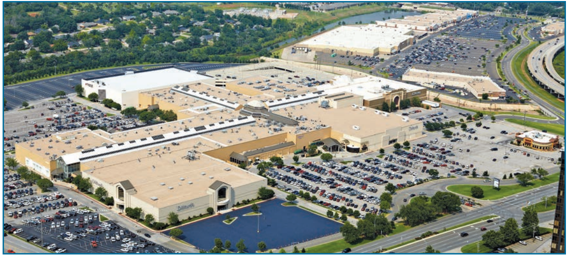
Photo 4 – The owner of this shopping mall chose BUR primarily due to its redundancy. Multiple plies of roofing can provide extra insurance against water intrusion.
