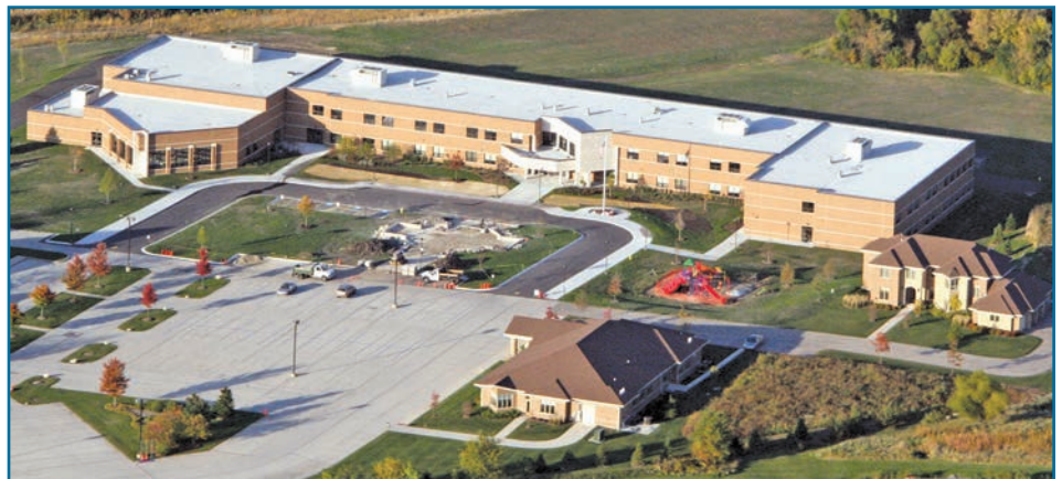
Photo 3 – The reflective roof on St. Patrick’s School, St. Charles, IL, was installed by Crowther Roofing & Sheet Metal, Romeoville, IL.
