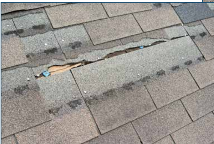
Figure 9 – Unnatural tear pattern from deliberate destruction.
