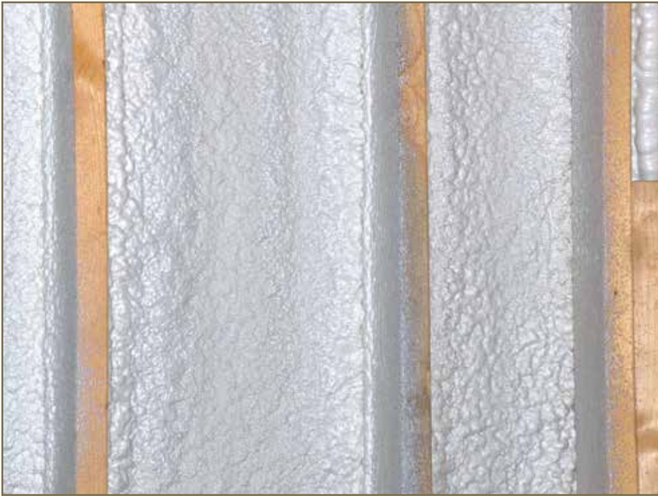
Photo 4 – Close-up of spray foam applied to walls.
