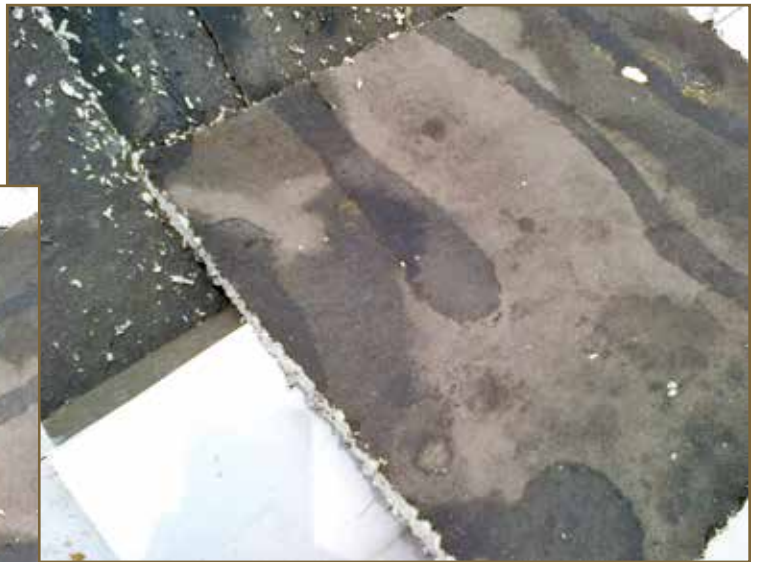
Photo 9 – Moisture between the layers of boards.
