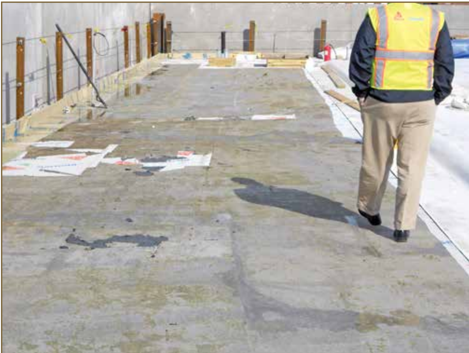
Photo 6 – Roofing removed from the perimeter.
