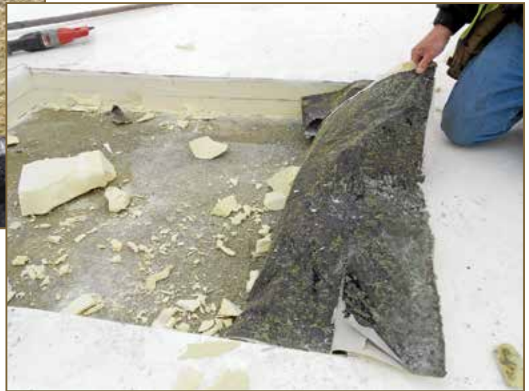
Photo 3 – Removal of adhered vapor barrier from primed concrete deck.
