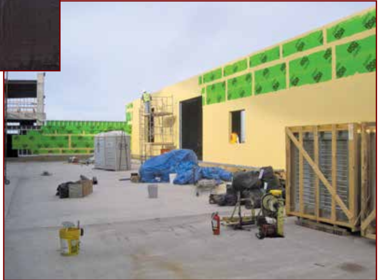
Photo 2 – Application of liquid-applied WRB.
