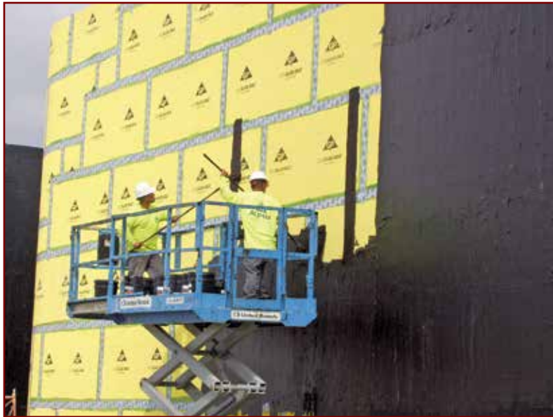
Photo 1 – Application of emulsion dampproofing.
