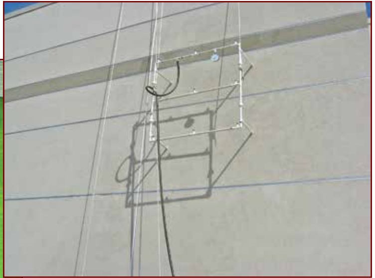
Photo 9 – Calibrated water spray rack on wall.
