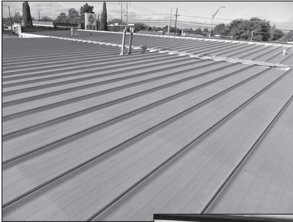
Figure 11 - 24-gauge metal roof installed in 1980.
