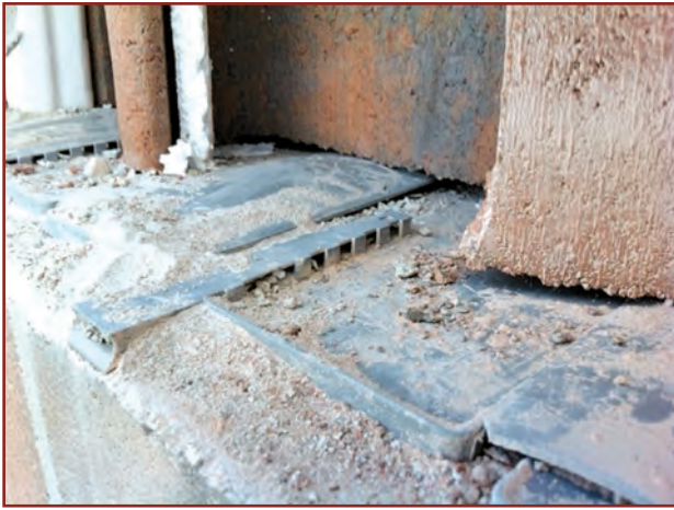
Figure 1 – Plastic pan flashing exposed in an investigation opening.
