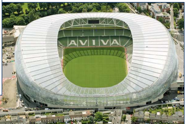
Figure 2 – Aviva football (soccer) stadium in Dublin, Ireland.
