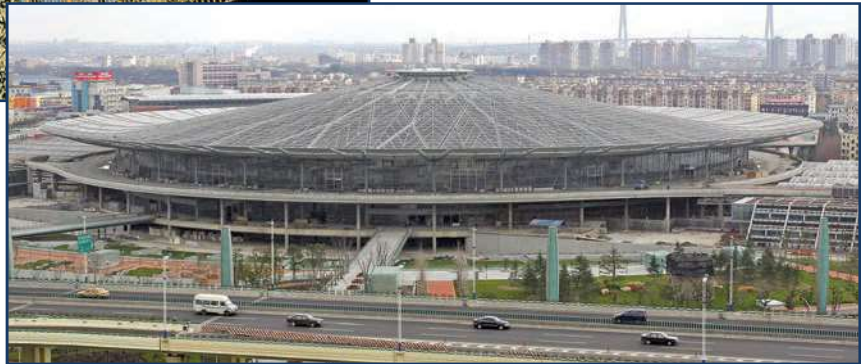
Figure 4 – The South Railway Station in Shanghai, China.
