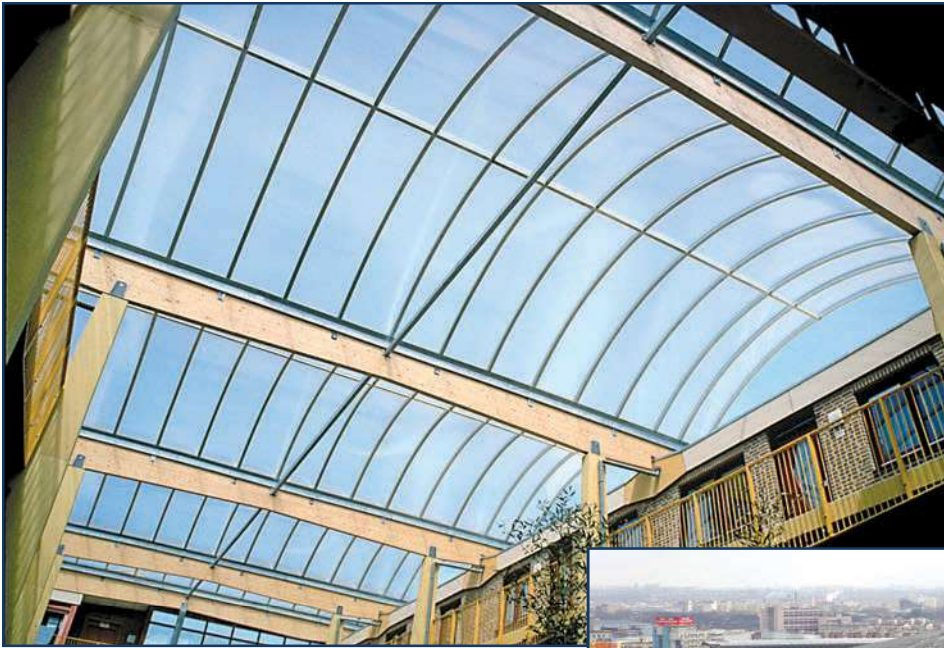
Figure 3 – An example of cold curving.
