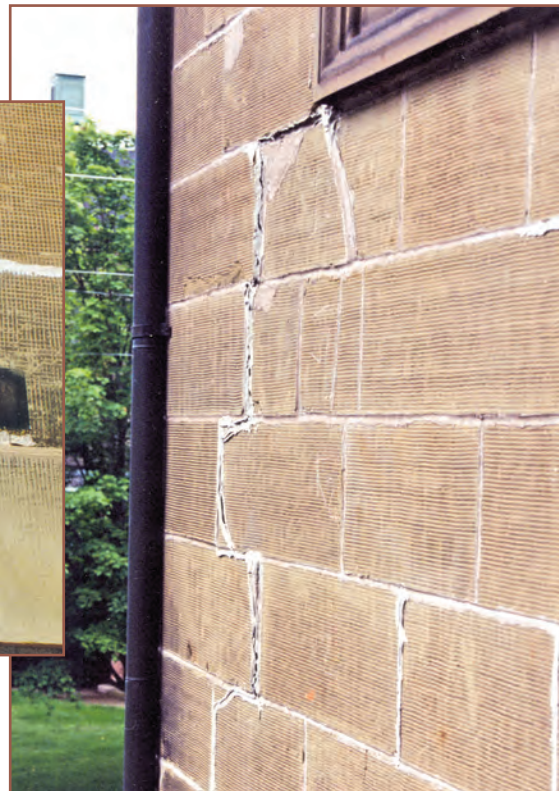
Figures 9 and 10 – Extensive cracking occurred after roof reconstruction work and many attempts at repair were carried out.
