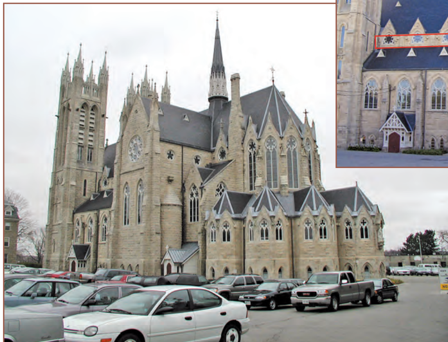
Figure 1 – Bowing of upper portions of the clerestory walls was first observed about ten years ago.
