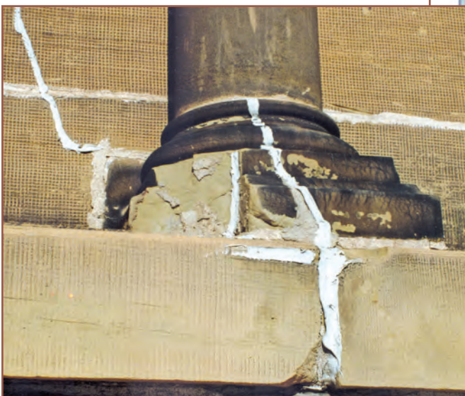
Figures 9 and 10 – Extensive cracking occurred after roof reconstruction work and many attempts at repair were carried out.
