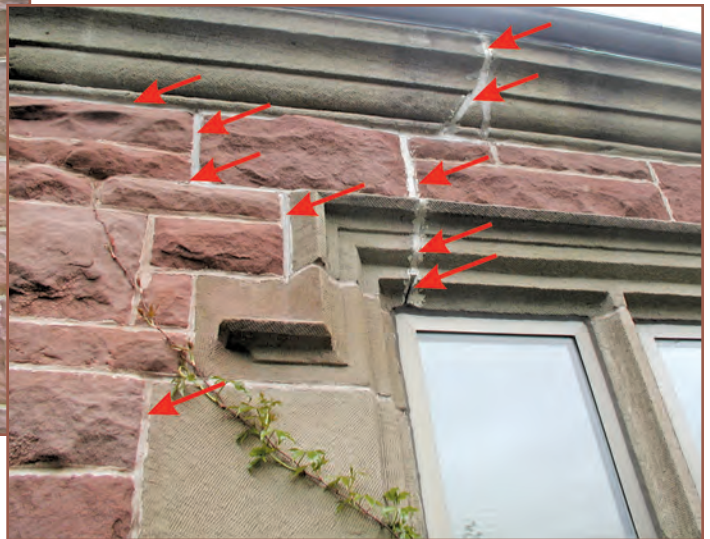
Figures 6 (left) and 7 (below) – Both of these buildings experienced extensive cracking following reroofing projects. Note the lintels rest only on the jambs. The building in Figure 6 also had hidden voids within its foundation walls.
