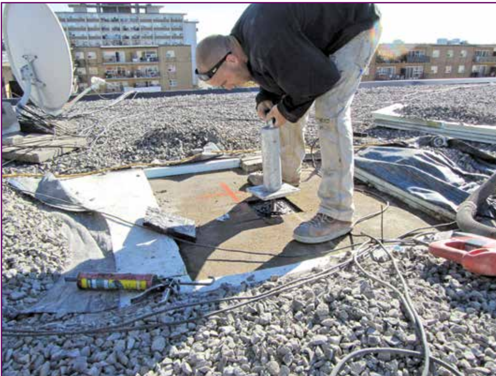
Figure 1 – Placing the roof anchor.
