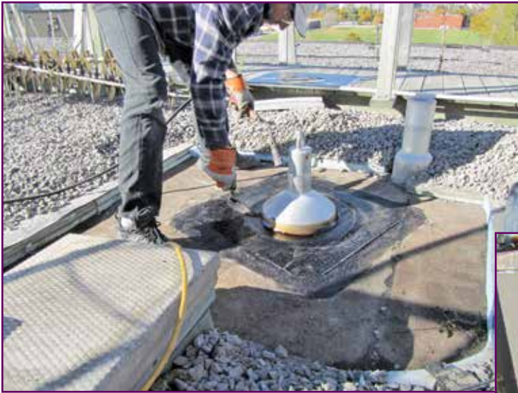
Figure 2 – Flashing the roof anchor.
