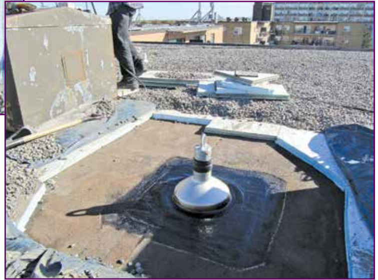
Figure 3 – Roof anchor patch completed.
